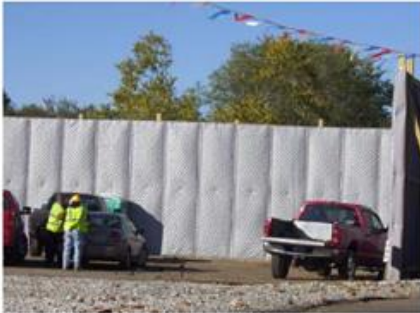
Figure 3 Substantial Temporary Construction Noise Barrier
