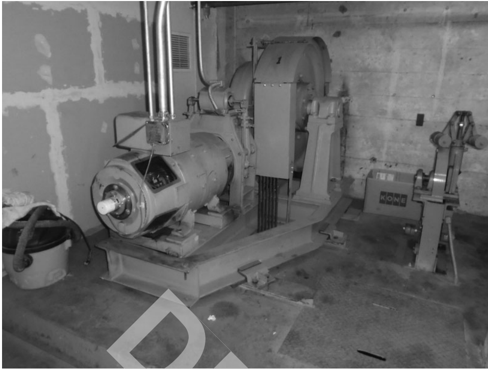
19. Traction elevator
