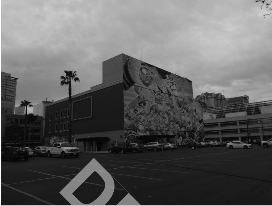
1. Subject property building at 300 S 1st St (with view of 4th floor mechanical area)
