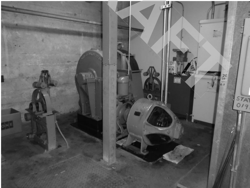
18. Traction elevator
