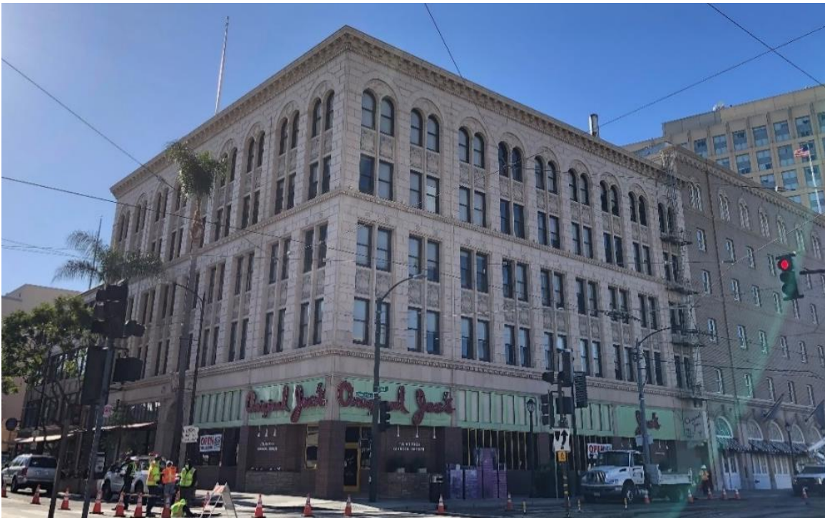
Photo 8: Surrounding development to the west.
