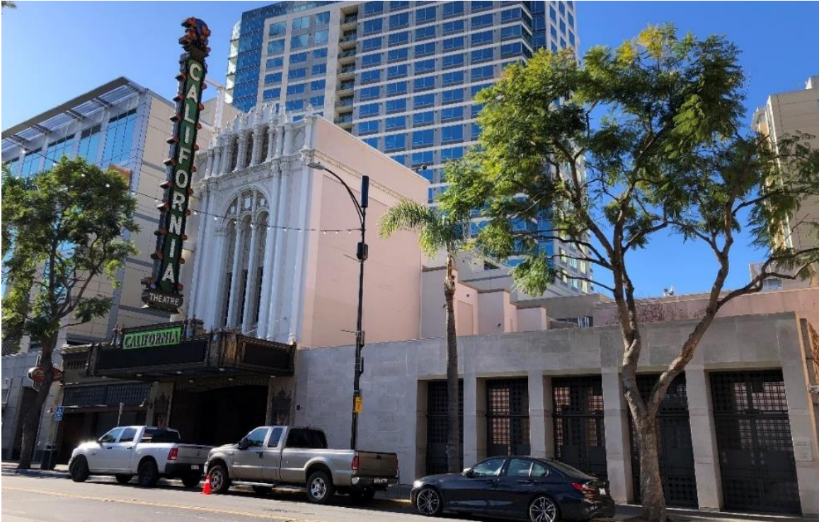
Photo 7: Surrounding development to the west.
