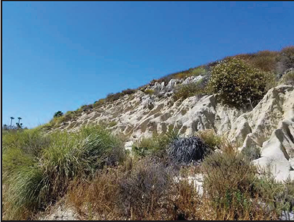
Photograph 8 – Looking Northwest – Slope Face Erosion near Park and Marina
