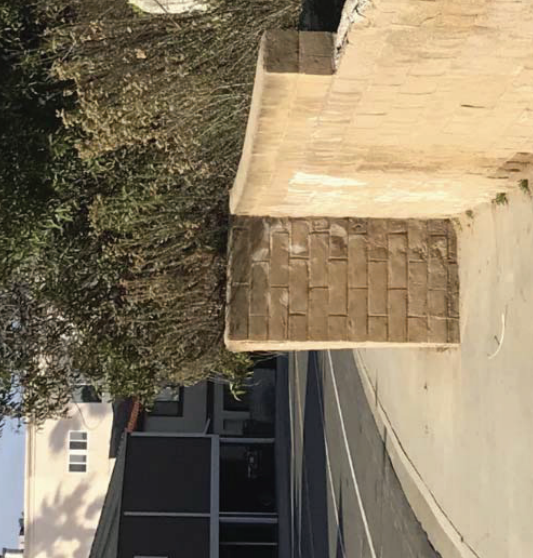
ABOVE: Sediment deposition after a December 2018 storm event BELOW: Portions of the retaining wall are beginning to lean toward the sidewalk
