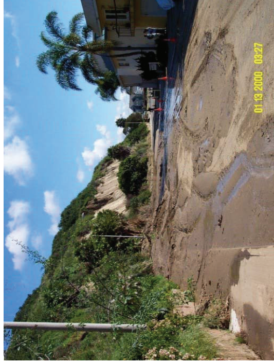
ABOVE: Degradation of the existing retaining wall BELOW: Sediment deposition after a January 2000 storm event
