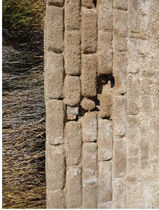
ABOVE: Degradation of the existing retaining wall BELOW: Sediment deposition after a January 2000 storm event
