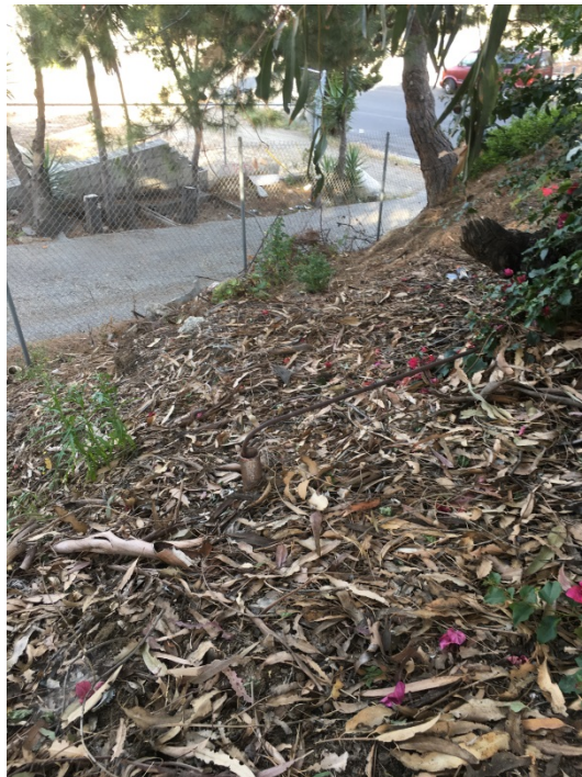
Photograph 4: Exposed vertical steel pipe on south central portion of Site, looking southwest.
