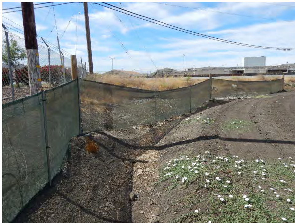
PP-11B Looking at confluence of multiple ditches discharging into roadside ditch.
