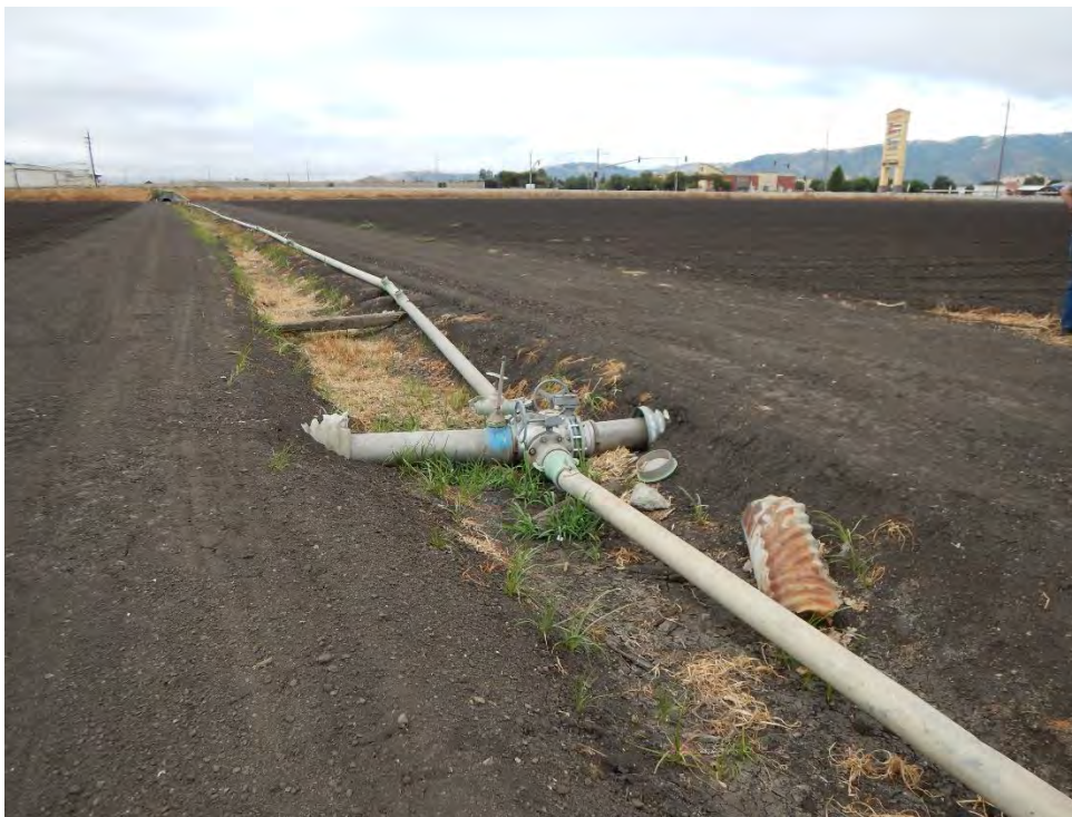
PP-7 Looking south along wetland swale at irrigation pipe junction.
