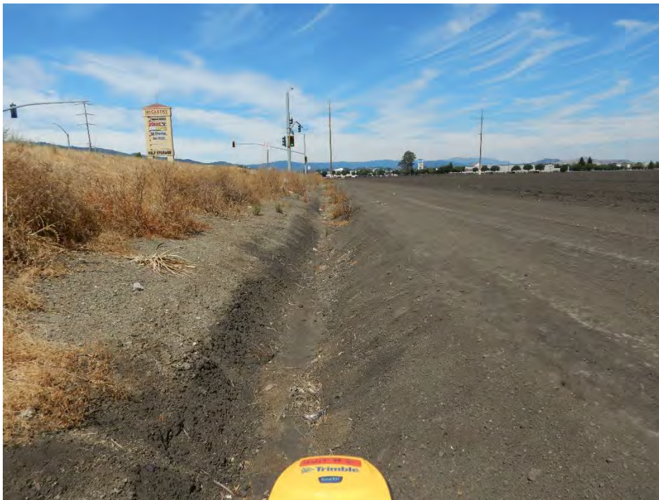
PP-10 Looking west up roadside ditch. Ends just before the light.
