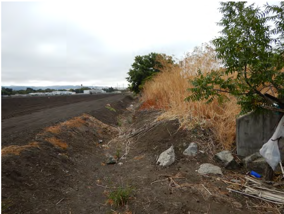
PP-9A Looking east up roadside ditch adjacent to large culvert.
