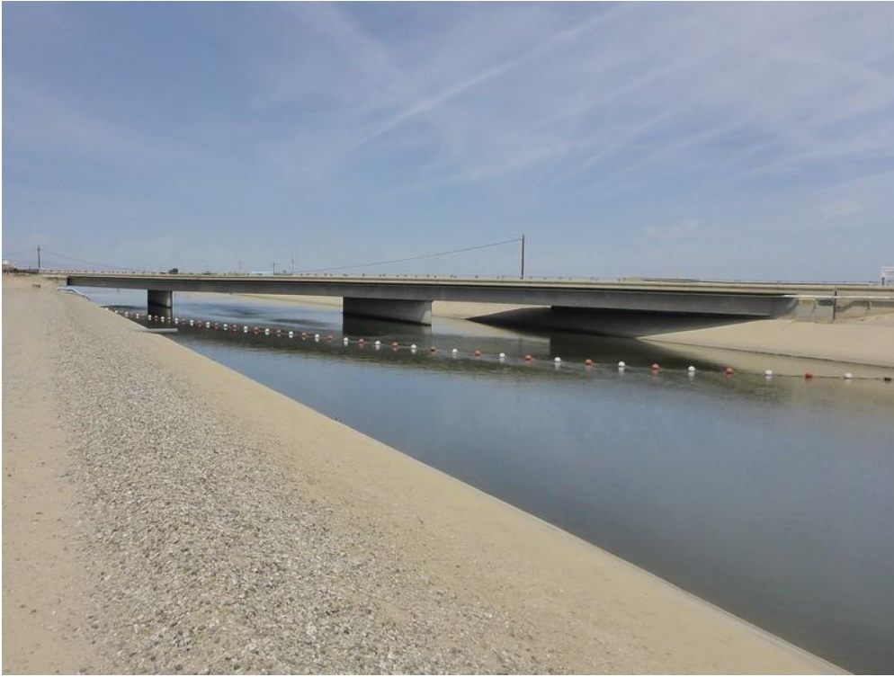
This is a wide shot of the existing bridge.
