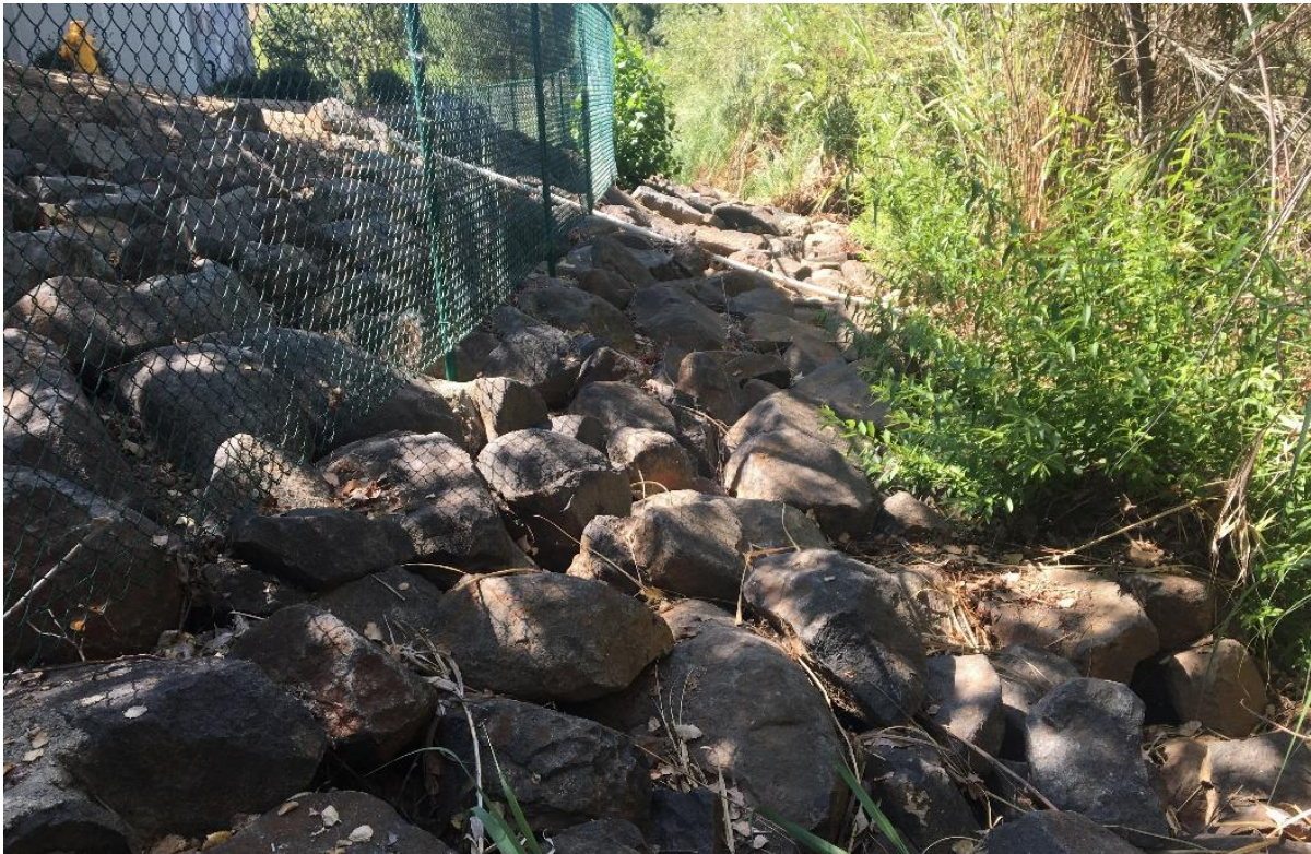
Figure 8 Eastern edge of project site, view south
