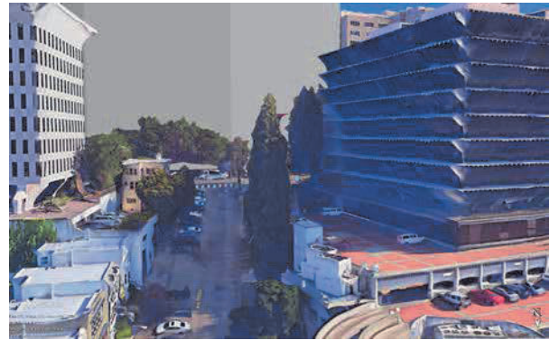
Figure 6 view south from Hill Point Way with new hospital
