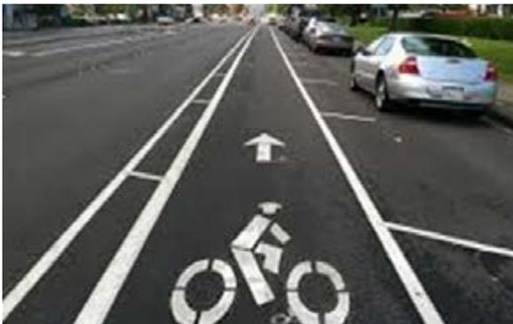
Class II: Bicycle Lane with a travel lane buffer and a parking lane buffer - Source: Kimley-Horn
