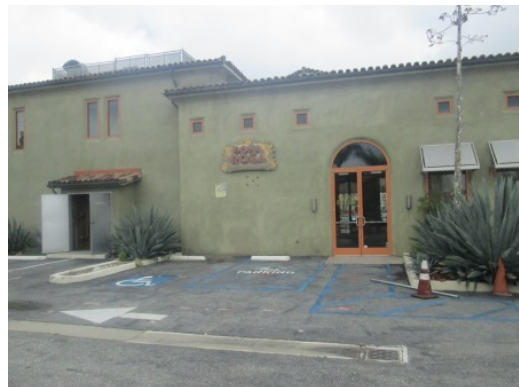
#30 WEST ELEVATION OF 577 BUILDING
