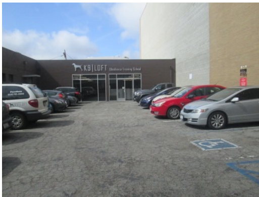
#11 NORTHWEST ELEVATION AND ASSOCIATED PARKING AREA OF 485-497 BUILDING (K9 LOFT)
