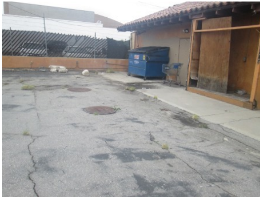
#61 BELOW-GRADE GREASE TRAP ON WESTERN EXTERIOR OF 541 BUILDING
