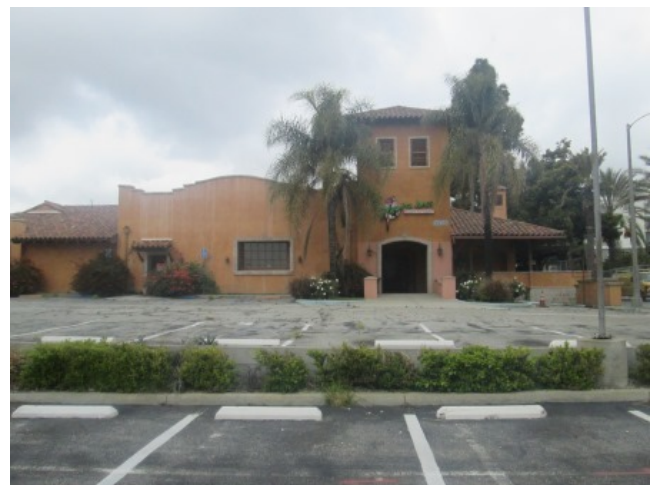
South elevation of 541 Building
