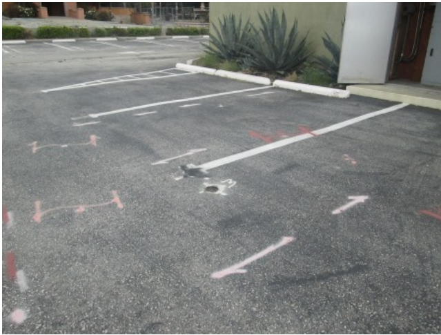
Evidence of former soil boring on western exterior of 577 Building
