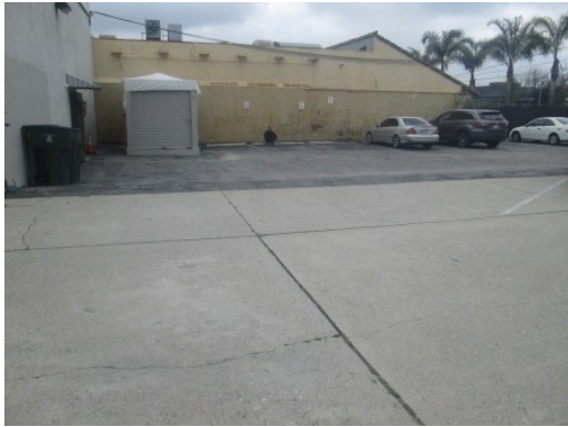
#21 PARKING AREA WEST OF 523 BUILDING
