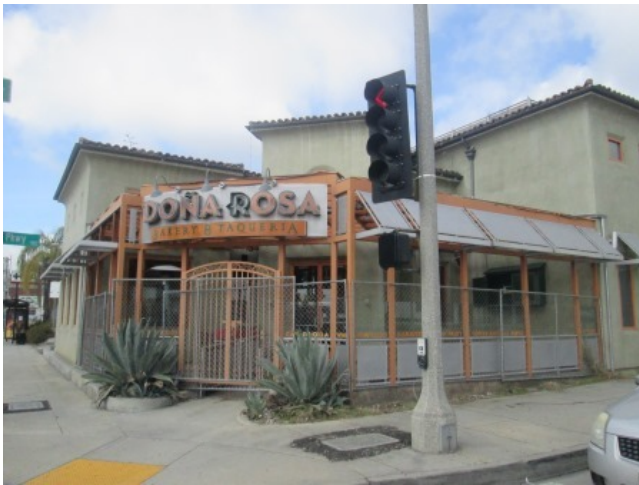
Southeast elevation of 577 Building
