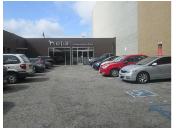
Northwest elevation and associated parking area of 485-497 Building (K9 Loft)
