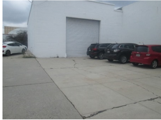
#14 SOUTHEAST ELEVATION OF 499/511 BUILDING
