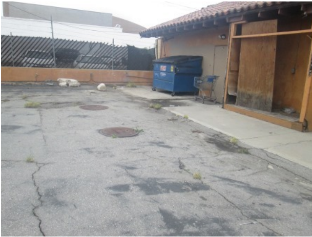
Below-grade grease trap on western exterior of 541 Building
