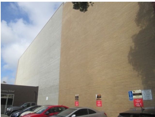
South elevation of 441-483 Building (Whole Foods)
