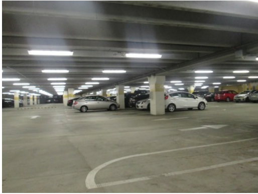
#37 WHOLE FOODS PARKING GARAGE (441-483)
