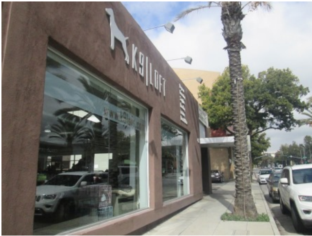
East elevation of 485-497 Building (K9 Loft)
