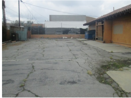
#26 PARKING AREA WEST OF 541 BUILDING
