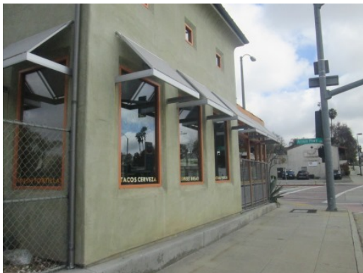
#29 SOUTH ELEVATION OF 577 BUILDING
