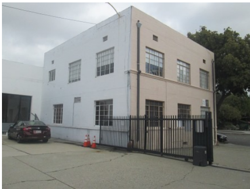
#17 SOUTHEAST ELEVATION OF 501 BUILDING
