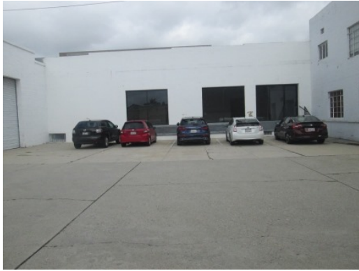
#13 SOUTH ELEVATION OF 499/511 BUILDING
