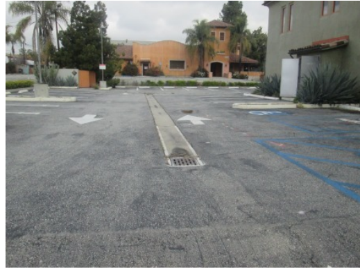
#32 PARKING AREA WEST OF 577 BUILDING
