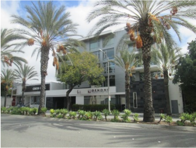
Adjacent east mixed-used building and Cisco Home store
