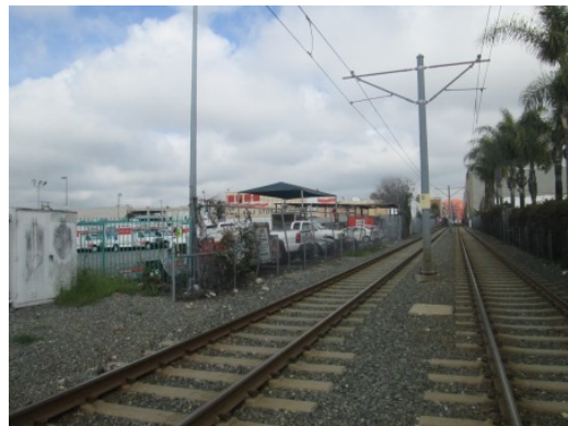
#78 ADJACENT WEST RAILROAD TRACKS AND U-HAUL FACILITY
