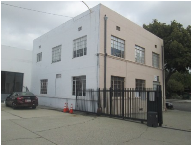
Southeast elevation of 501 Building
