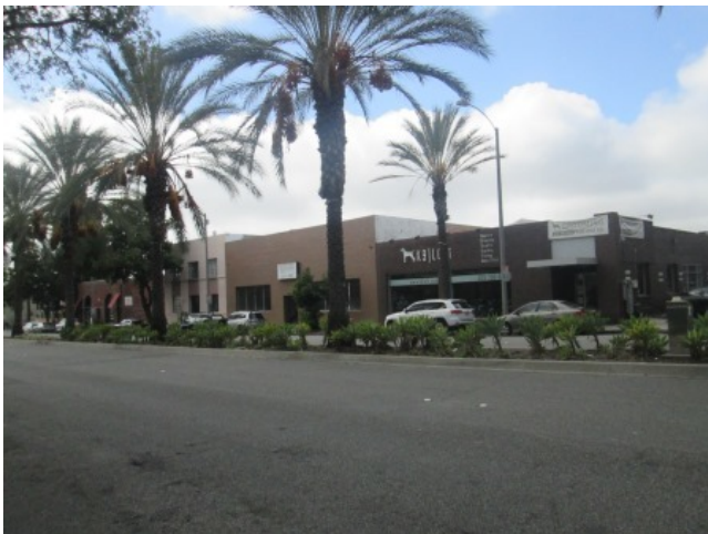
East elevation of Project
