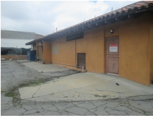
West elevation of 541 Building
