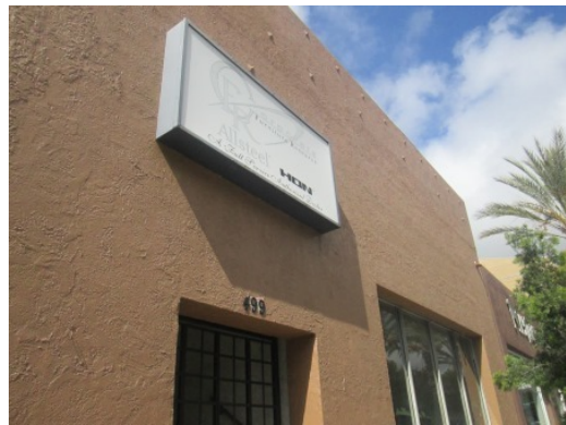
#12 EAST ELEVATION OF 499/511 BUILDING
