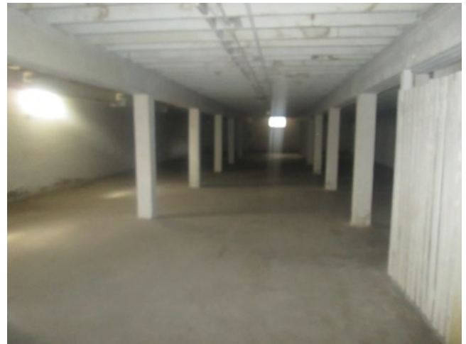
499/511 Building basement interior
