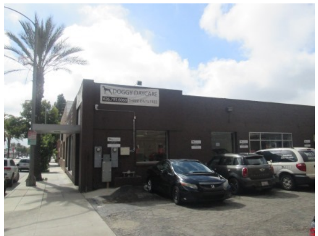
Northeast elevation of 485-497 Building (K9 Loft)
