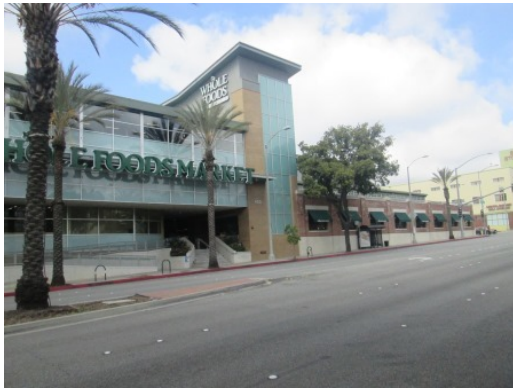
#7 EAST ELEVATION OF 441-483 BUILDING (WHOLE FOODS)
