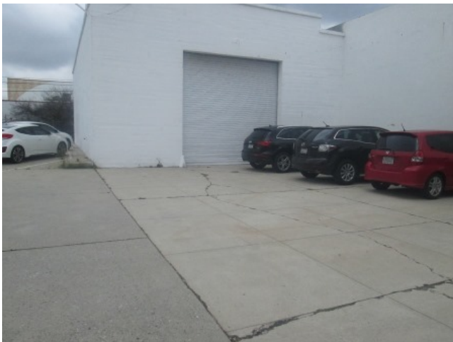
Southeast elevation of 499/511 Building
