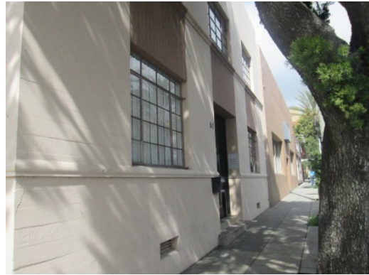
#16 EAST ELEVATION OF 501 BUILDING
