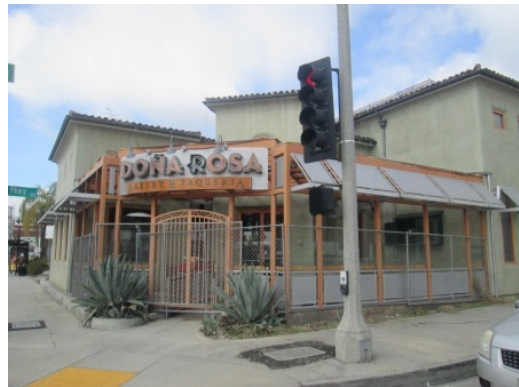
#28 SOUTHEAST ELEVATION OF 577 BUILDING
