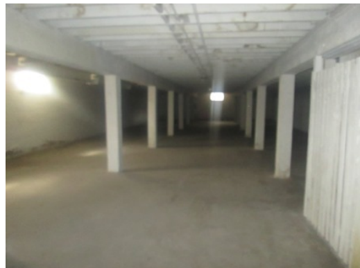
#42 499/511 BUILDING BASEMENT INTERIOR
