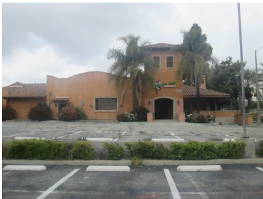
#23 SOUTH ELEVATION OF 541 BUILDING
