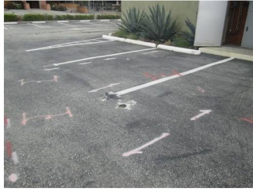
#68 EVIDENCE OF FORMER SOIL BORING ON WESTERN EXTERIOR OF 577 BUILDING
