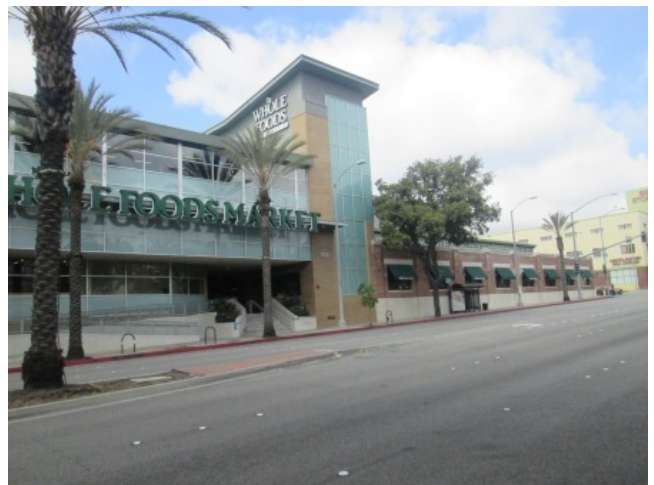
East elevation of 441-483 Building (Whole Foods)
