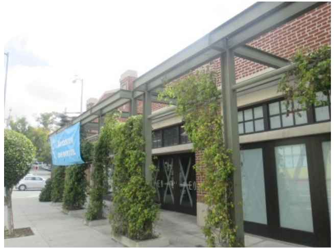
Northeast elevation of 441-483 Building (Whole Foods)
