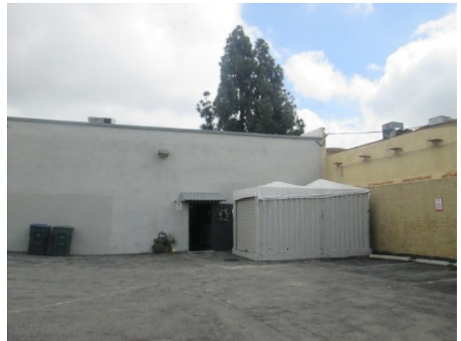
West elevation of 523 Building
