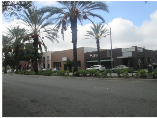
#2 EAST ELEVATION OF PROJECT
