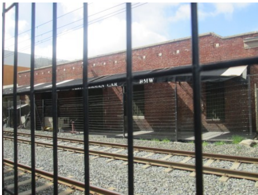
#77 ADJACENT WEST RAILROAD TRACKS AND PLATI GERMAN CAR SERVICE
