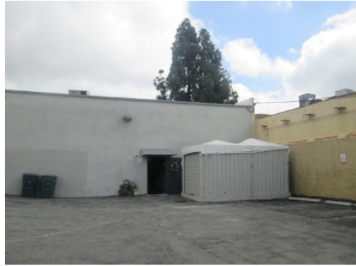
#20 WEST ELEVATION OF 523 BUILDING
