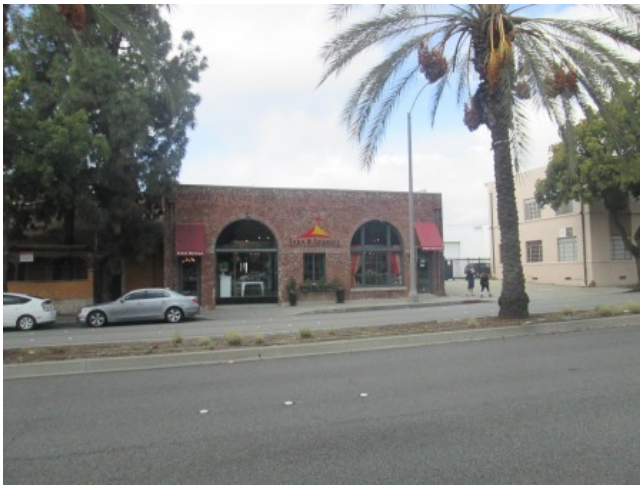
East elevation of 523 Building
