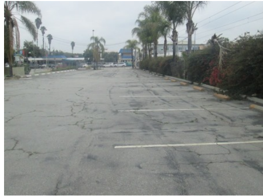
#34 PARKING AREA ON WEST-SOUTHWEST PORTION OF PROJECT
