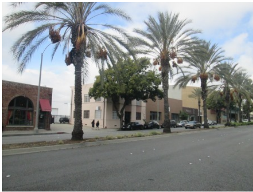
#3 EAST ELEVATION OF PROJECT
