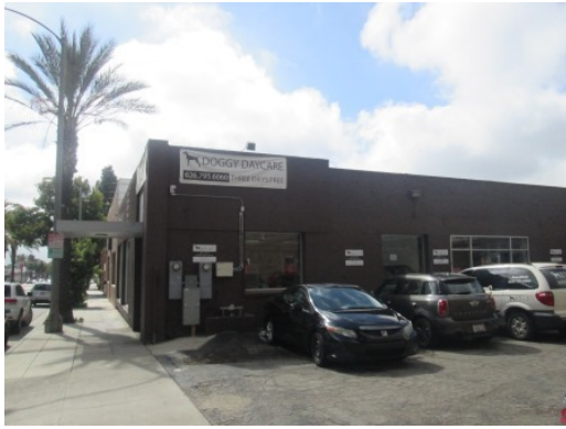
#9 NORTHEAST ELEVATION OF 485-497 BUILDING (K9 LOFT)
