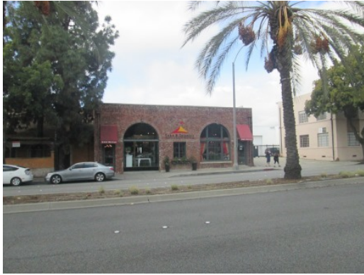
#19 EAST ELEVATION OF 523 BUILDING
