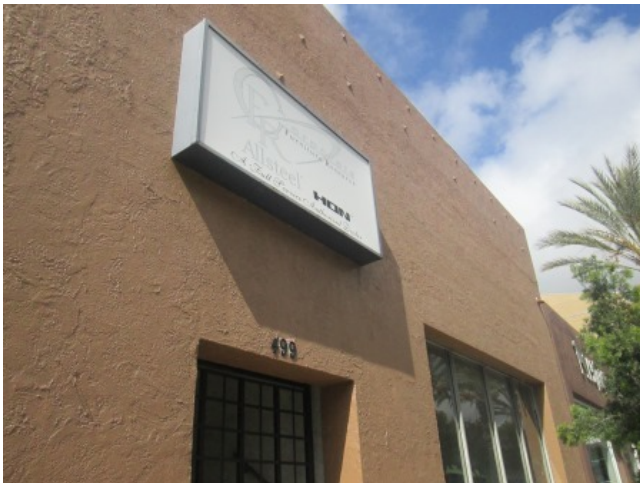
East elevation of 499/511 Building
