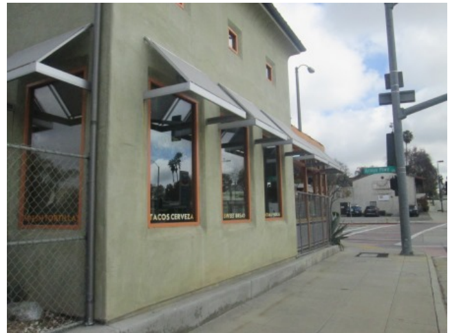
South elevation of 577 Building
