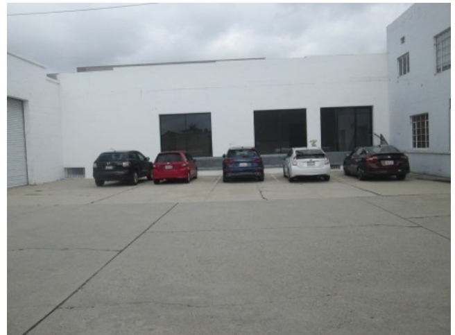
South elevation of 499/511 Building
