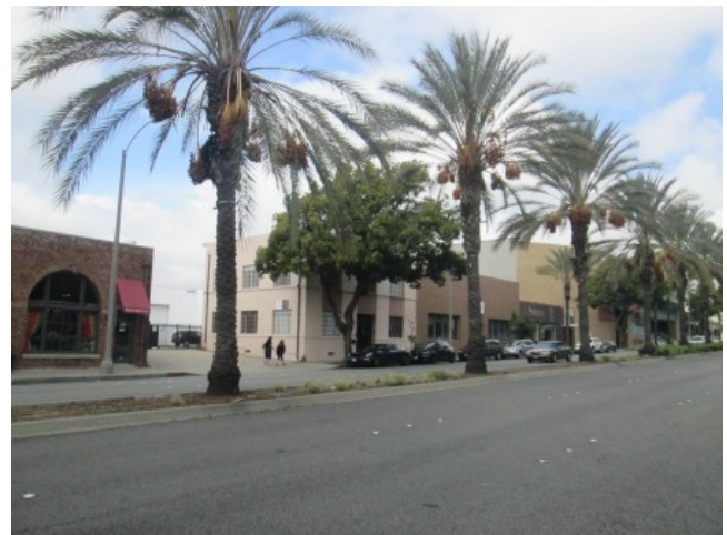
East elevation of Project
