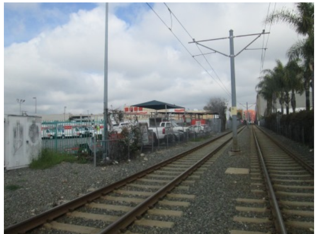
Adjacent west railroad tracks and U-Haul facility
