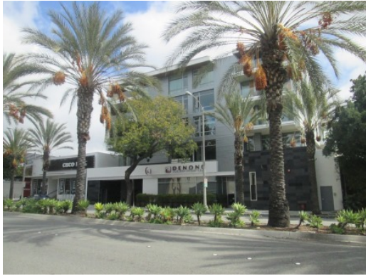
#73 ADJACENT EAST MIXED-USED BUILDING AND CISCO HOME STORE
