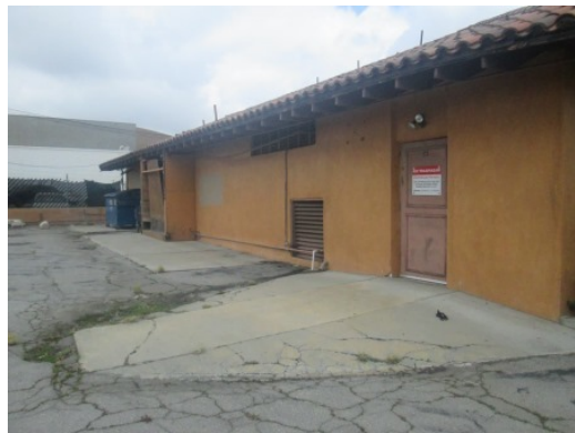
#24 WEST ELEVATION OF 541 BUILDING
