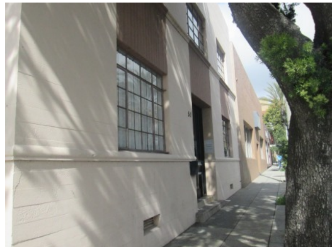
East elevation of 501 Building
