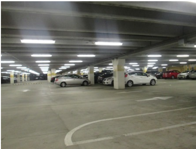
Whole Foods parking garage (441-483)
