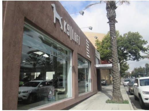
#10 EAST ELEVATION OF 485-497 BUILDING (K9 LOFT)
