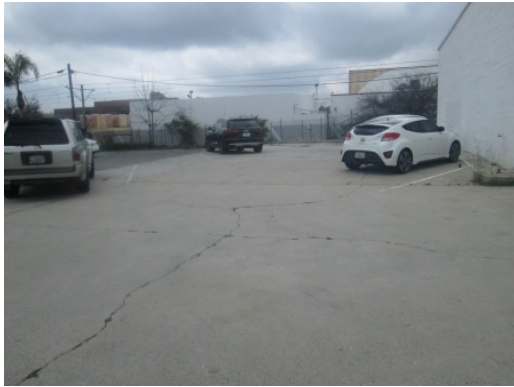
#15 PARKING AREA SOUTH OF 499/511 BUILDING (APPROXIMATE LOCATION OF FORMER "GASOL PUMP")
