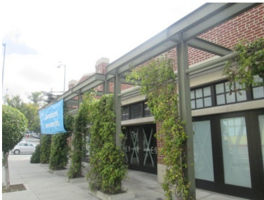
#5 NORTHEAST ELEVATION OF 441-483 BUILDING (WHOLE FOODS)
