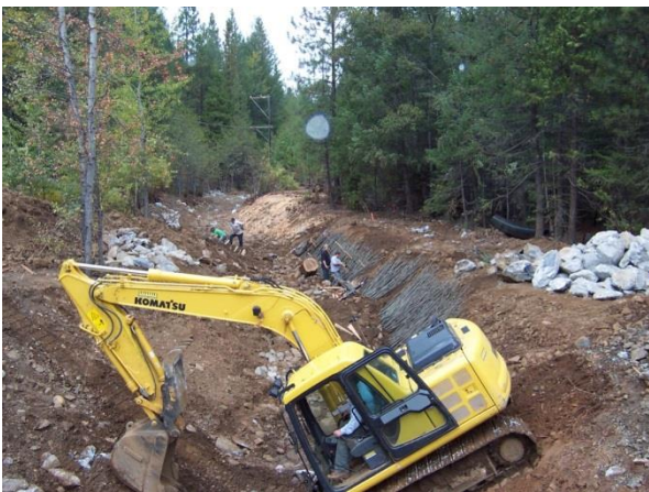
Figure 7-6: Construction of grade control veins into the banks and below channel grade (note: grade control boulders and willow plantings materials in background).
