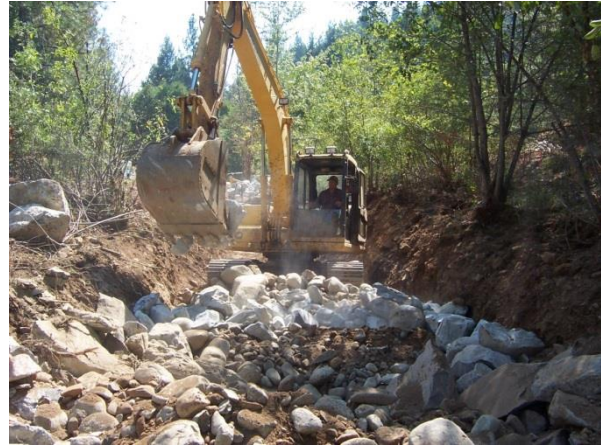
Figure 7-5: Installation of stream bed materials.
