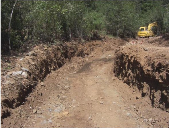
Figure 7-4: A section of Little Browns Creek dewatered, aggraded materials removed and excavation below the channel grade in order to install streambed materials and grade control structures. The excavation provided mechanical access to the stream reach.
