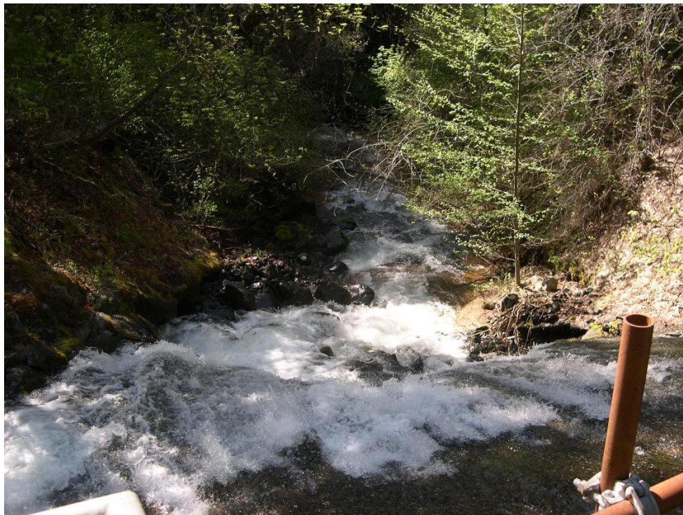
ii: East Weaver Dam- photo taken from the intake structure near the crest of the dam, looking downstream.
