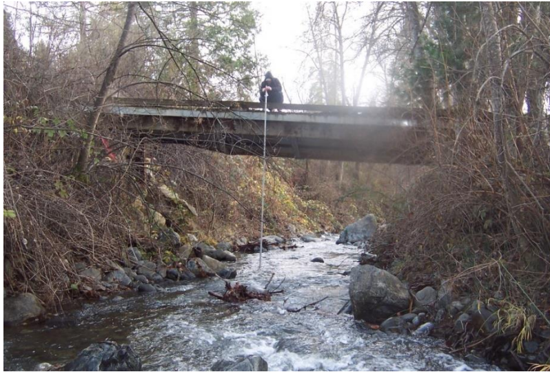
Figure 10-8: Bonar Private Road Bridge in December 2015.
