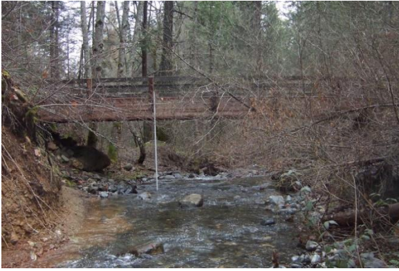
Figure 10-2: East Weaver Campground Pedestrian Bridge Spans the entire floodplain of East Weaver Creek.
