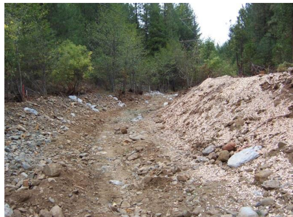
Figure 7-7: Grade control veins are buried every 25' and the channel bottom bedload materials in place (final jetting and washing fines has not been done at this stage).
