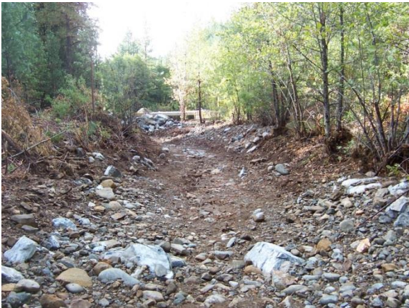
Figure 7-10: Channel with grade structures buried and channel bottom before final jetting.
