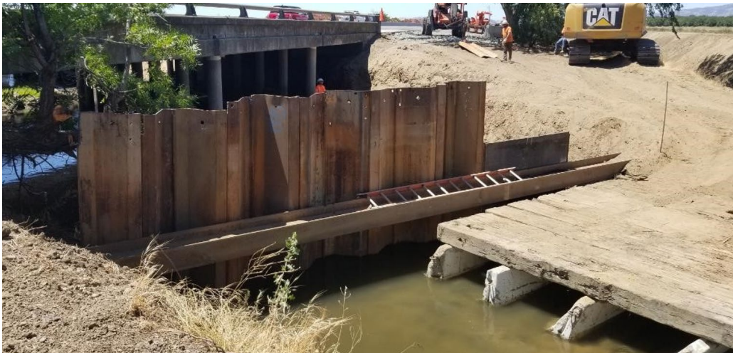
Photo 8: A typical timber mat built out of 8-inch-thick timbers.
