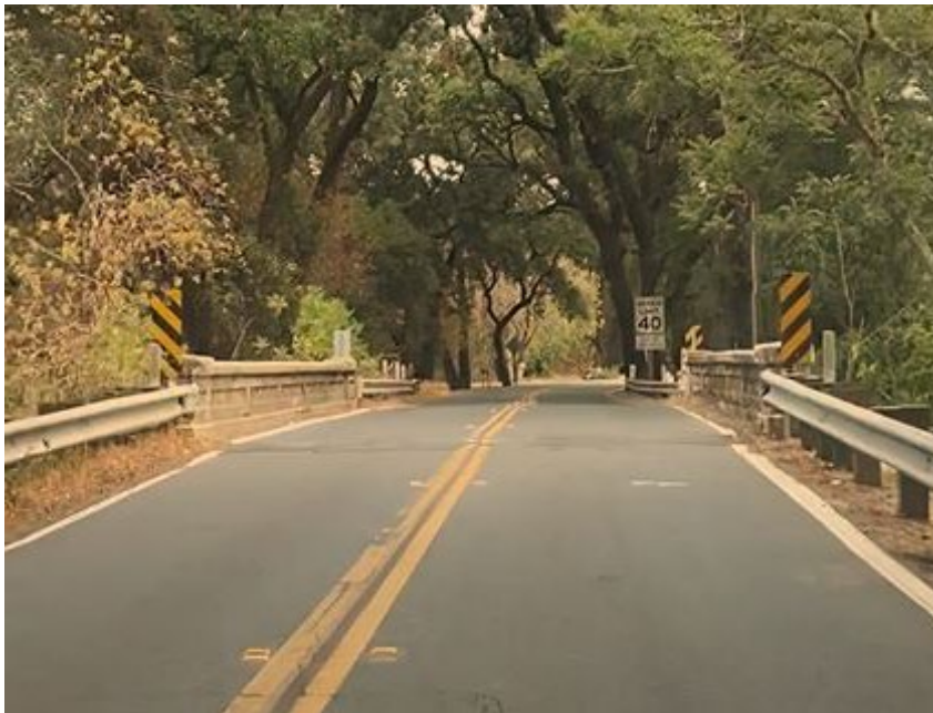
Photo 1: Looking eastbound toward Hopper Slough Bridge displaying MBGR, no shoulders, and 10-foot-wide travel lanes (taken in 2021).
