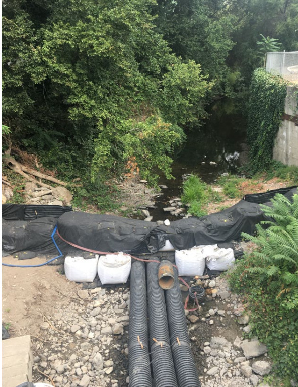
Photo 7: Example of typical temporary creek diversion – Cofferdam.
