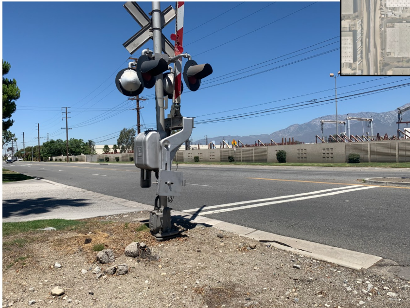
View 2: South of the Project Site, at the intersection of Slover Ave. and Union Pacific Railroad, looking Northwest.
