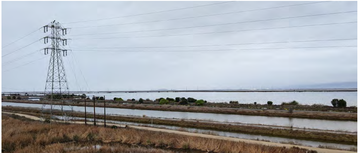
Electrical infrastructure along Sunnyvale Bay Trail
