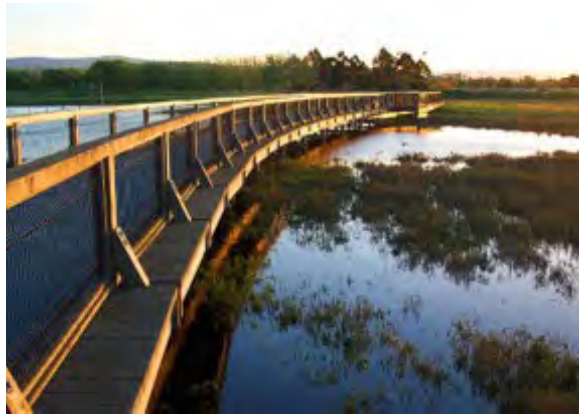
Bridge over waterway
