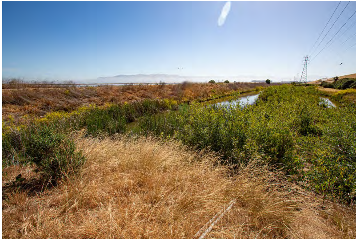
Cleanwater Construction Project; looking east along the channel in the forebay system; stormwater detention channel
