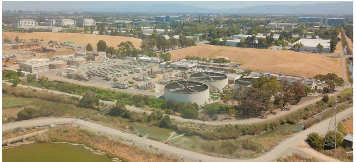
"Sunnyvale Water Pollution Control Plant from the air" by Grendelkhan, licensed under CC BY-SA 4.0
