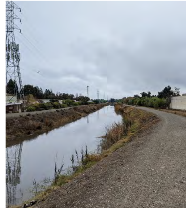
View along East Channel
