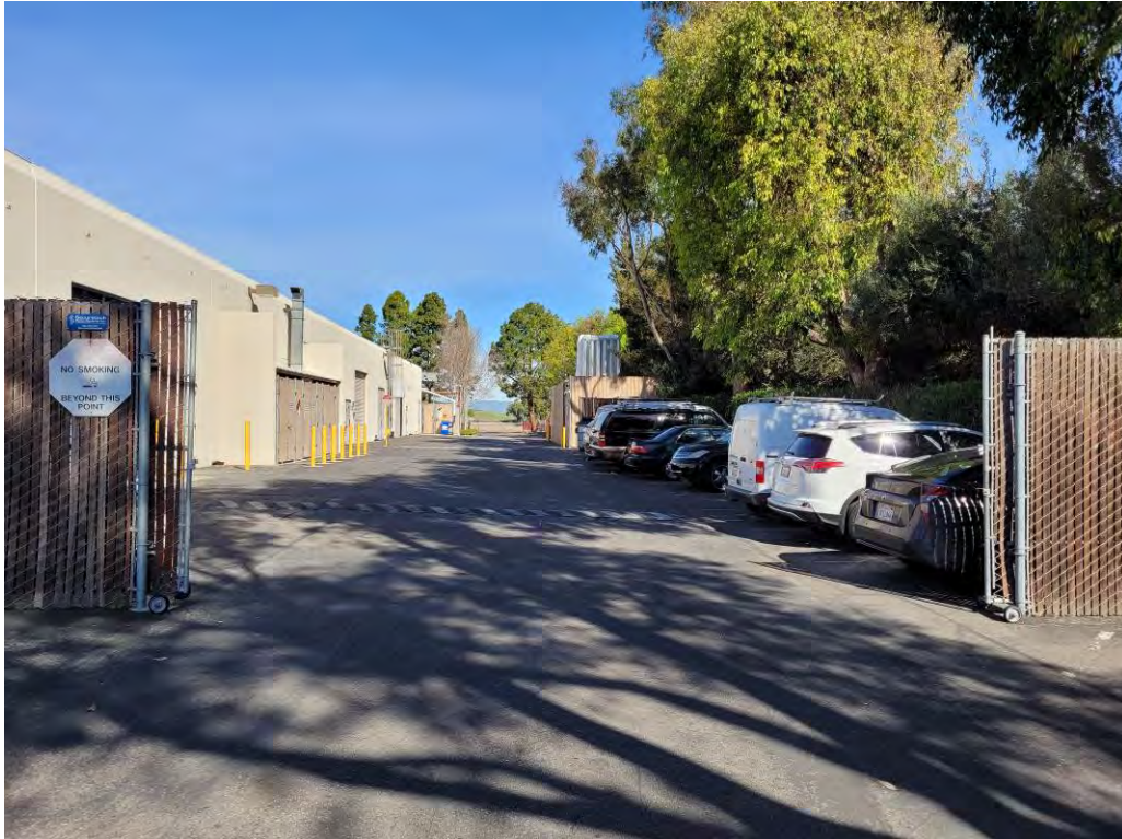
Photograph 5: 1320 Bordeaux Drive, enclosures possibly associated with a groundwater treatment system.
