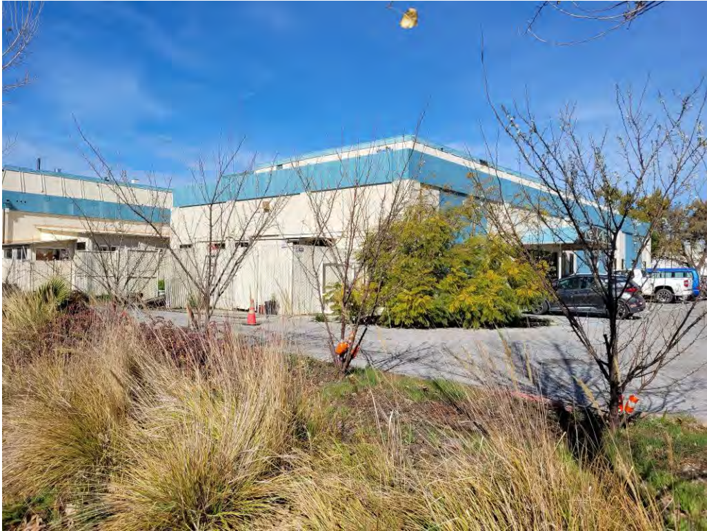
Photograph 3: 1230 Bordeaux Drive, possible groundwater treatment system enclosure.
