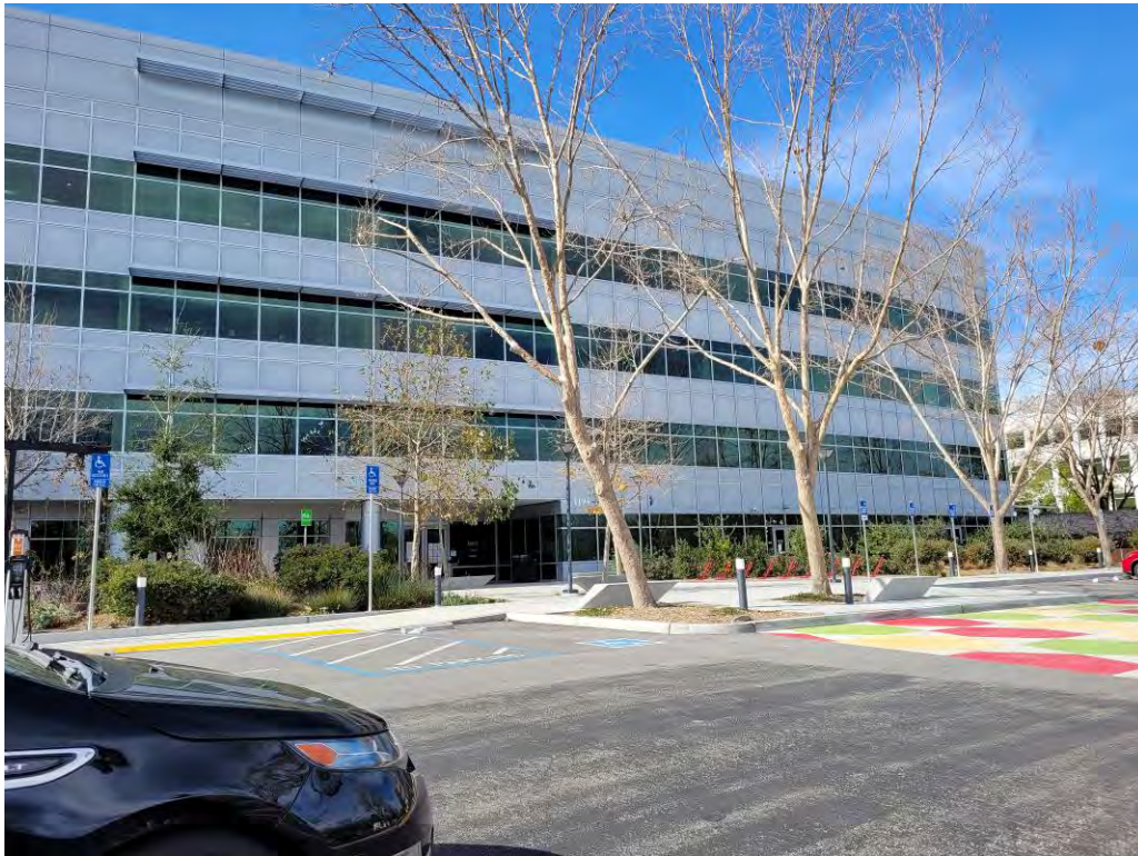
Photograph 2: 1194 North Mathilda Avenue, Google Building 1194.
