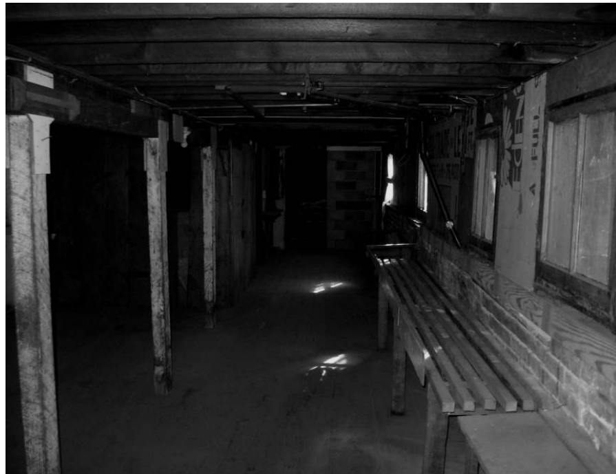
Photo 35: View of basement, note fruit drying tables.
