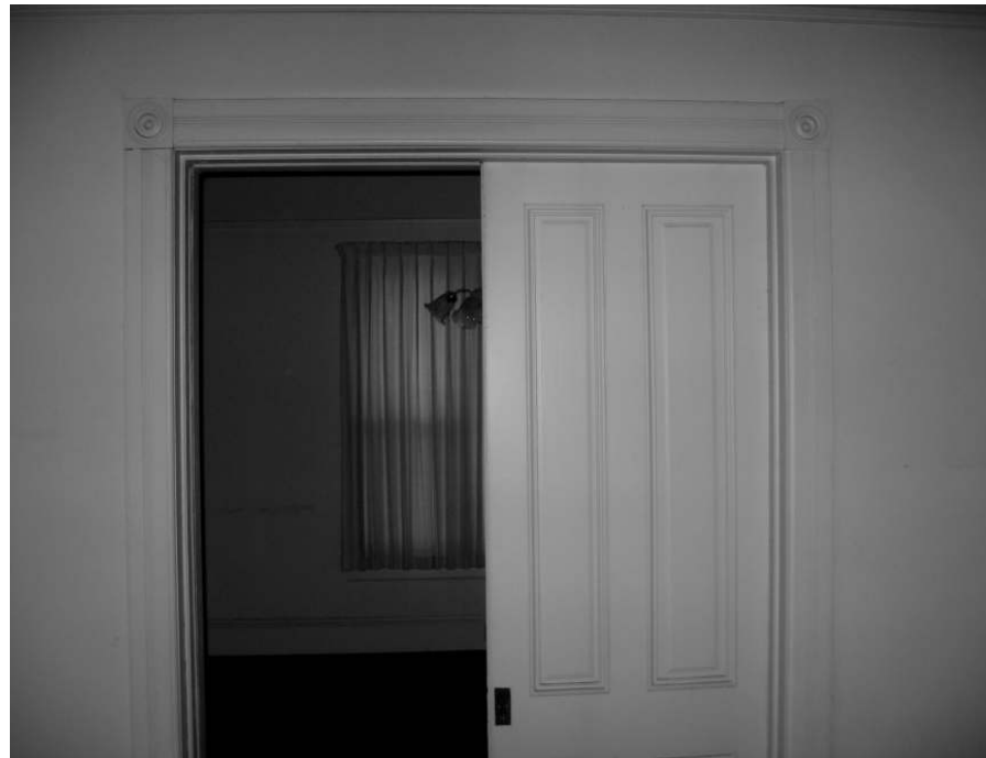
Photo 23: View of partially closed pocket doors.
