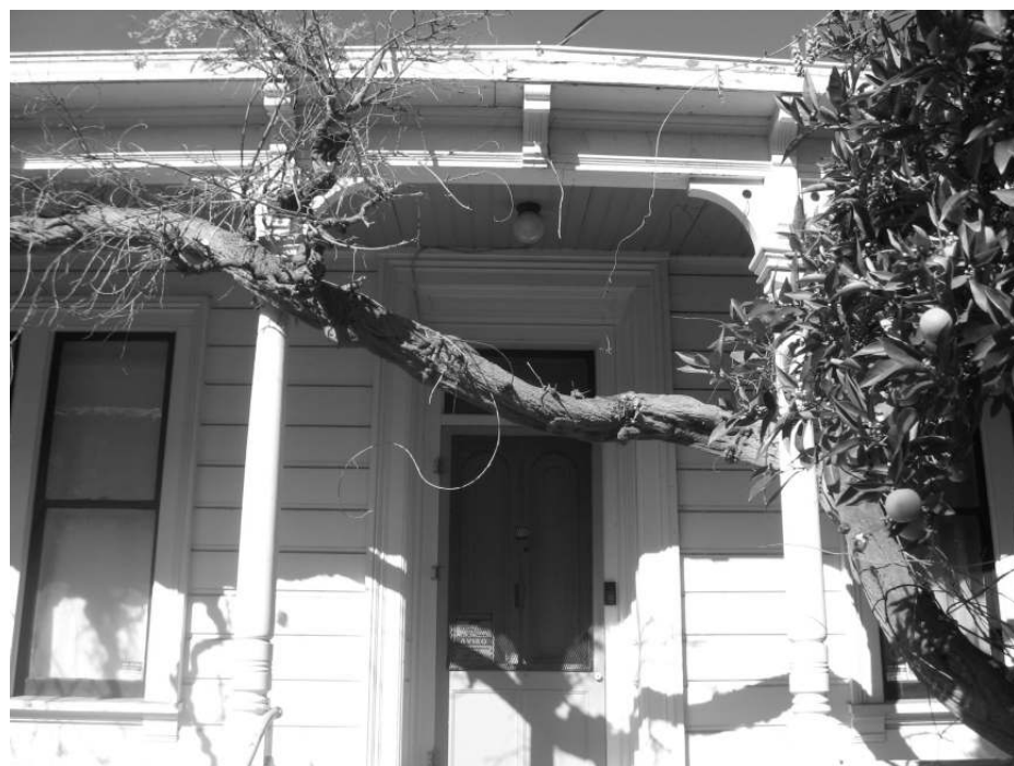
Photo 2: View of the entry and front porch.
