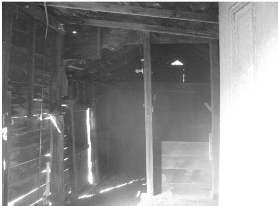
Photo 42: Interior view of the tank house.
