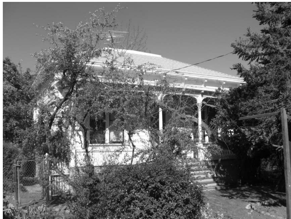
Photo 1: View of the front facade of 1065 S. Winchester Blvd.
