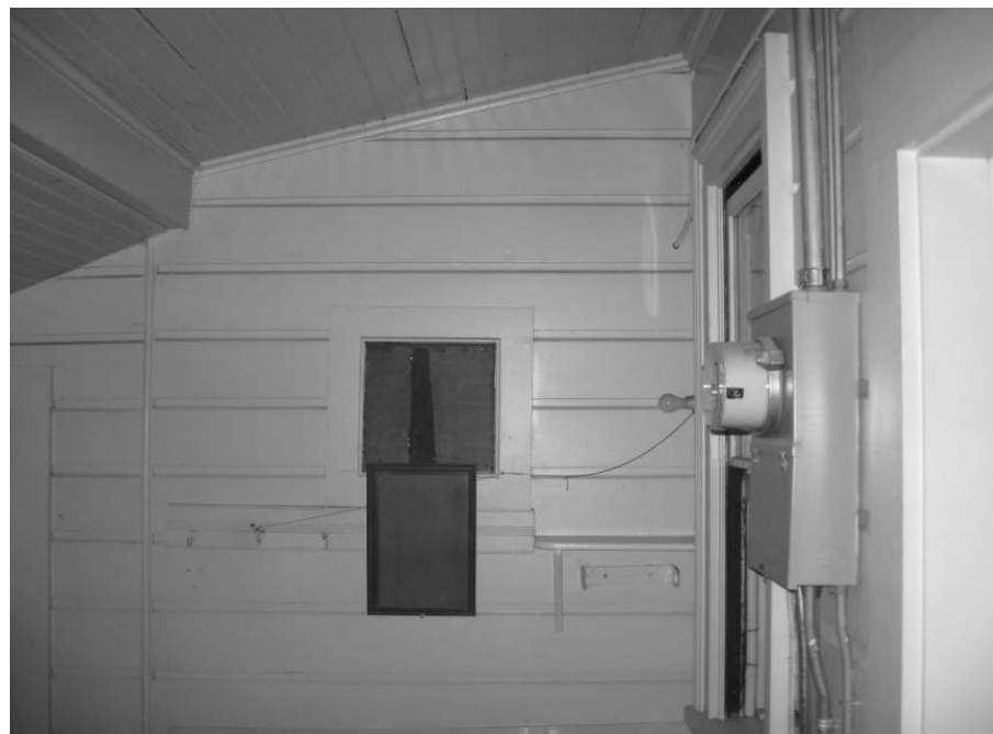
Photo 30: View of the interior of the utility/mud room, rear addition.
