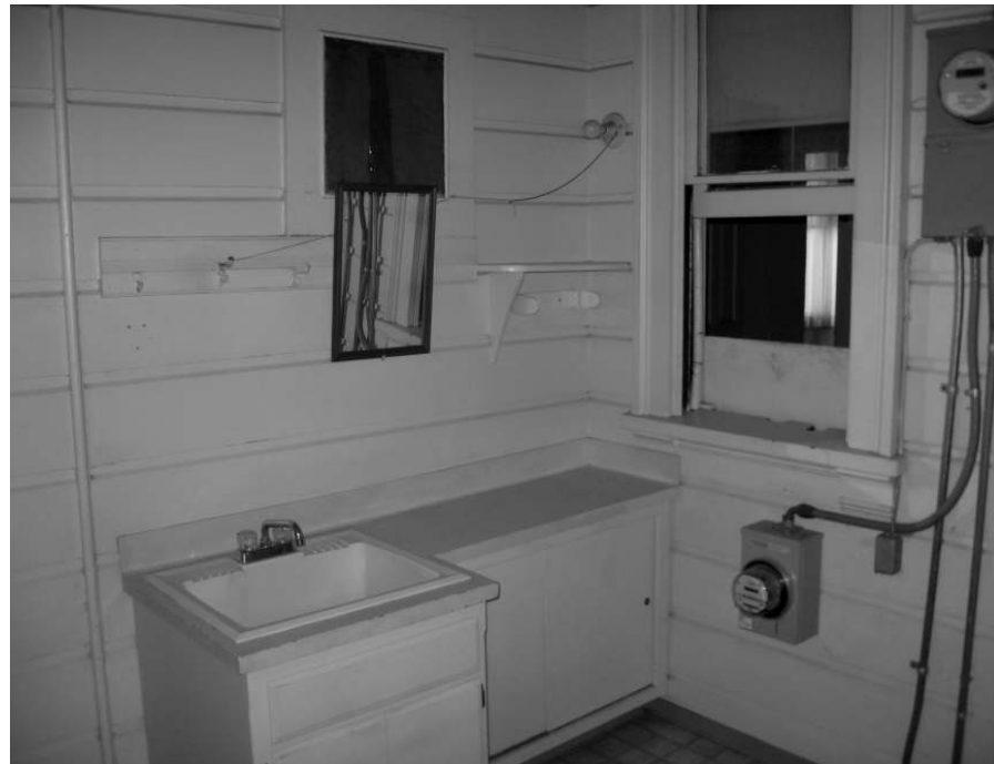
Photo 31: Another view of the utility/mud room.
