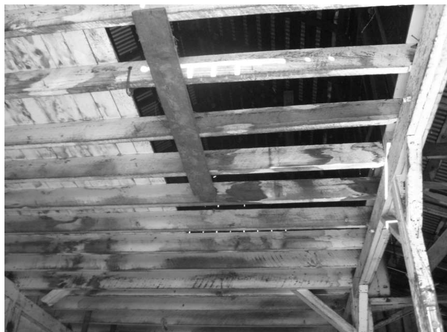
Photo 52: View up into hay loft area of the barn.
