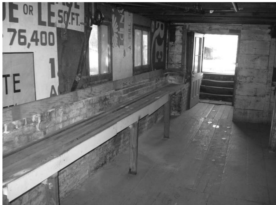
Photo 36: View of basement showing drying tables, brick foundation.
