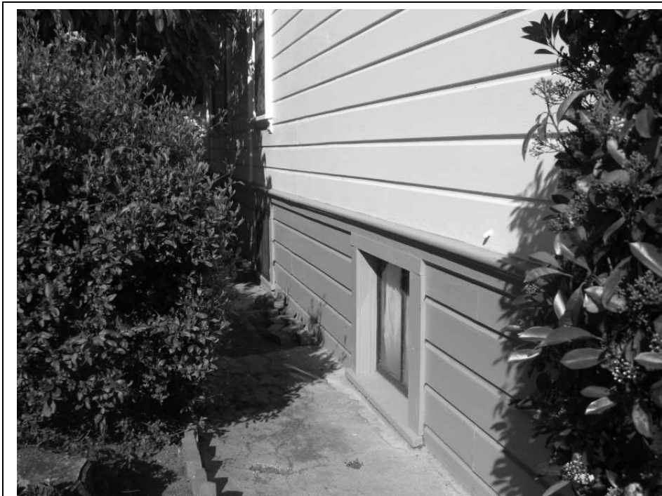
Photo 9: View along the southern facade.
