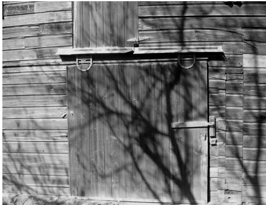
Photo 49: View of the central, sliding door of the barn.
