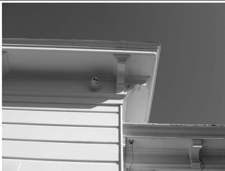
Photo 8: Detail of boxed and enclosed eaves with decorative brackets.
