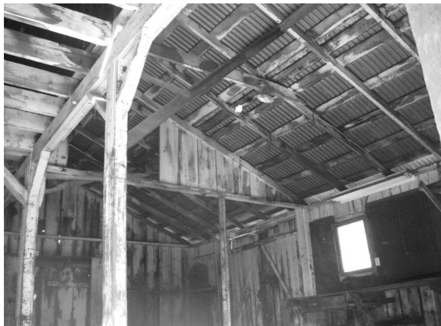
Photo 50: View of the interior of the barn.
