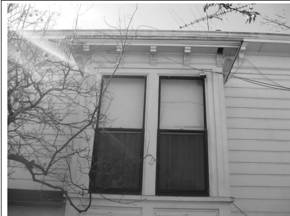
Photo 14: Detail of extending bay on the northern facade.
