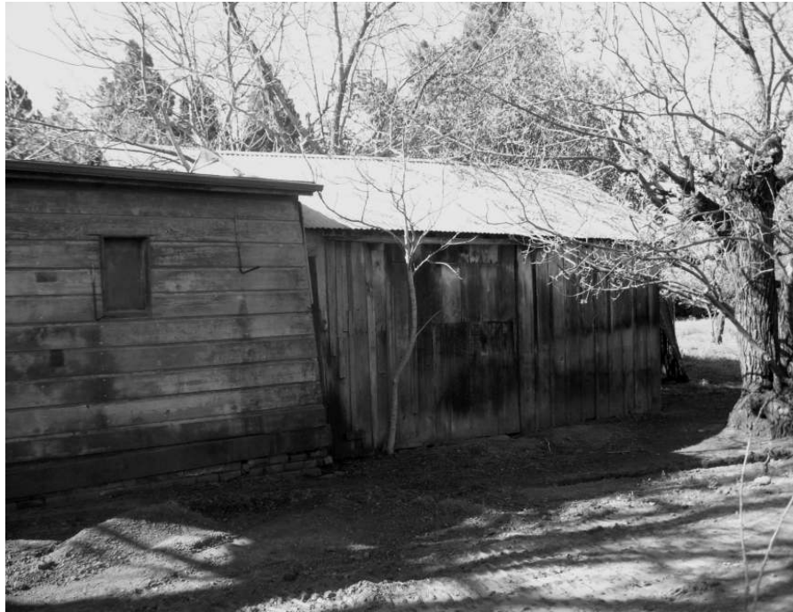
Photo 41: View of the shed addition from the north.
