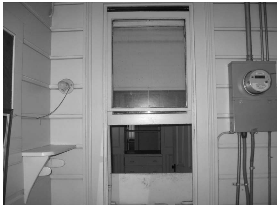
Photo 32: Detail of original rear facade window in rear addition.
