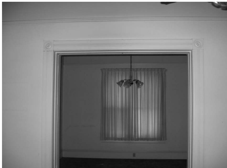
Photo 22: View of pocket doors in dining room.
