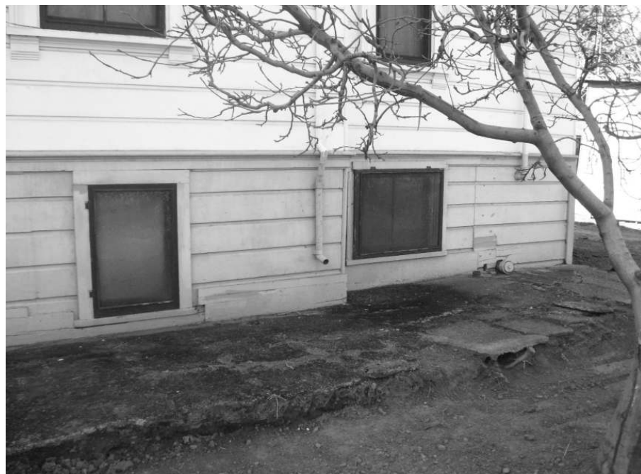
Photo 16: View of basement level windows on the northern facade.
