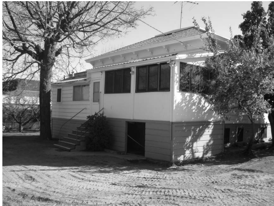
Photo 11: oblique view of the rear facade showing additions.
