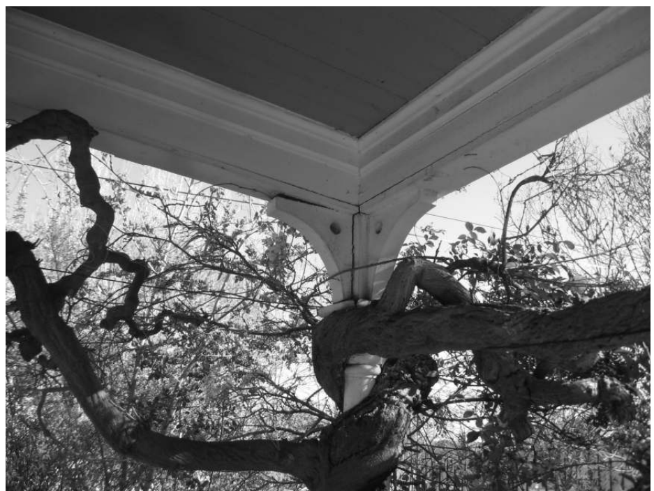
Photo 6: Detail of support column and braces on the front porch.
