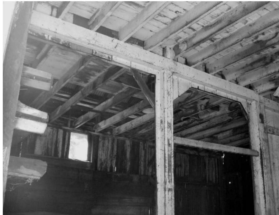
Photo 51: Another view of the interior on the barn showing trusses.
