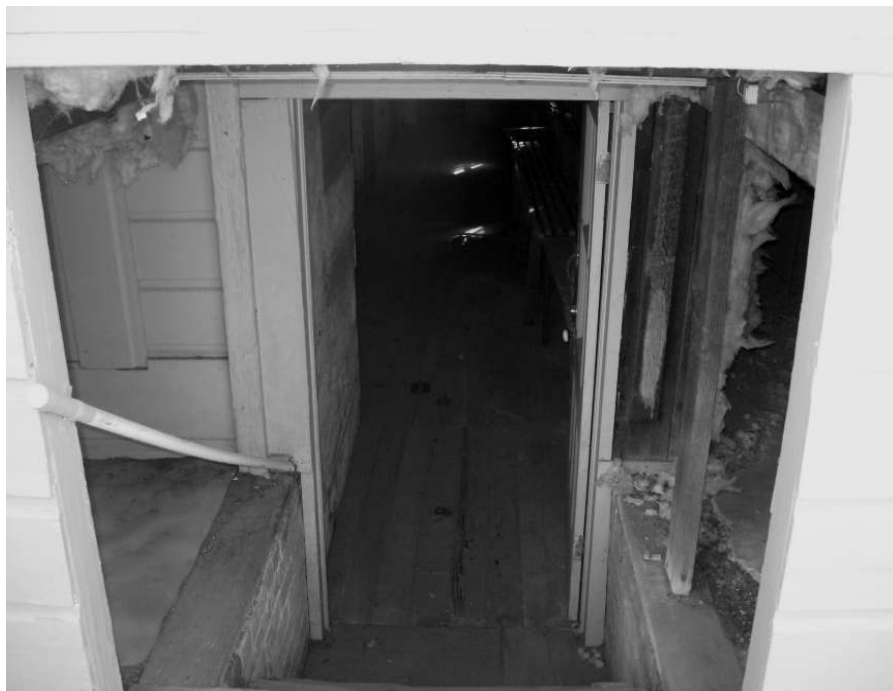
Photo 33: View down basement entry steps on rear facade.
