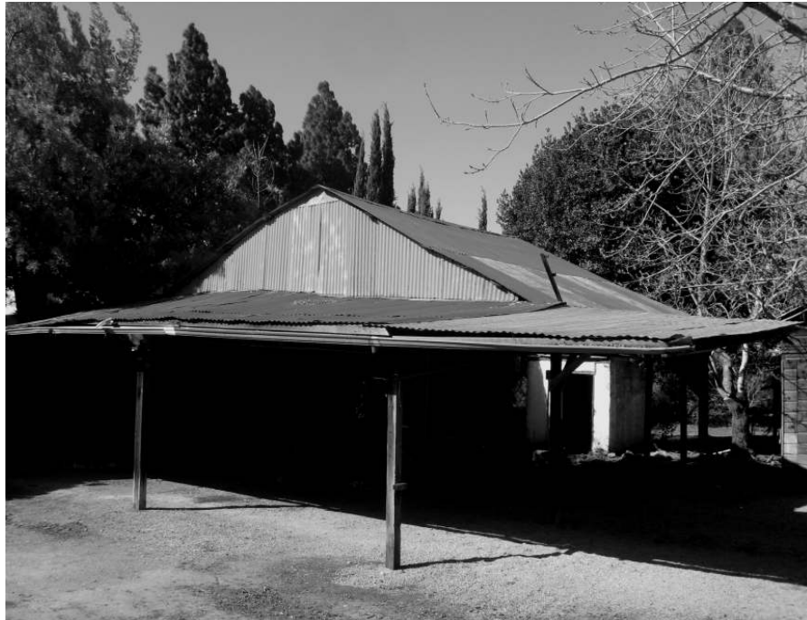
Photo 53: View of covered fruit-drying area.
