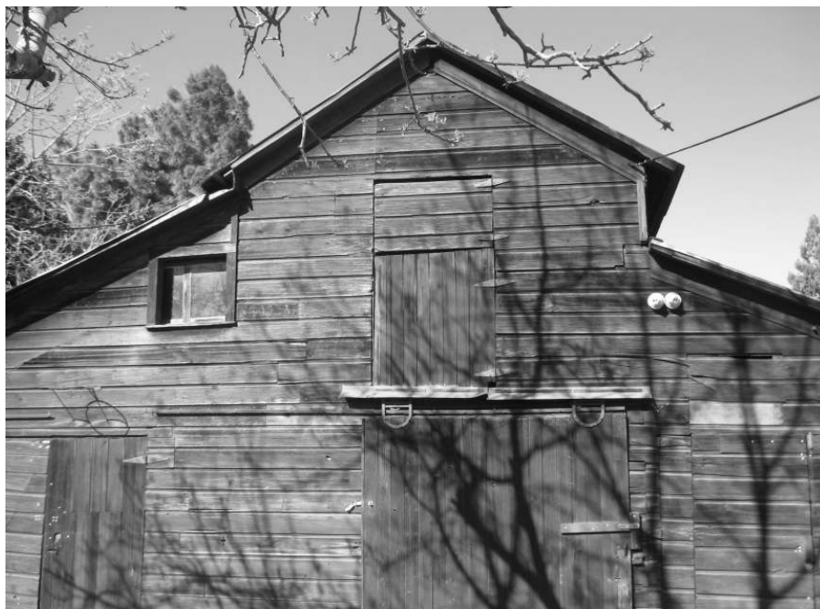
Photo 44: A closer view of the front facade of the barn.
