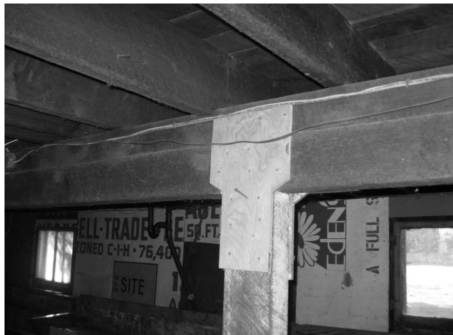
Photo 38: View of support beam in the basement.
