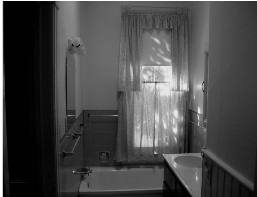
Photo 29: View of the bathroom. Note non-original fixtures.
