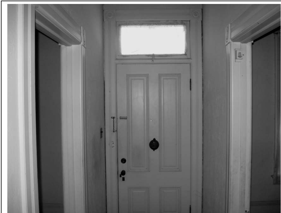
Photo 17: Interior view of the front entry, note transom window.
