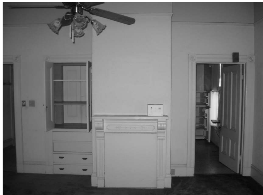
Photo 20: View of covered fireplace and mantel.
