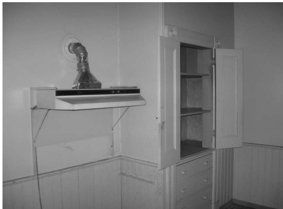
Photo 28: Another view of the kitchen, showing pass-through cabinet.
