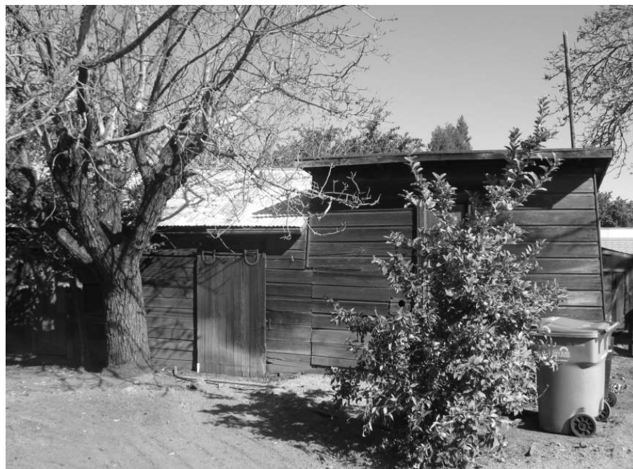
Photo 40: View of tank house from the south showing shed addition.
