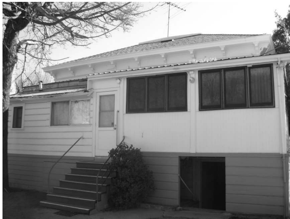
Photo 12: View of the rear additions.
