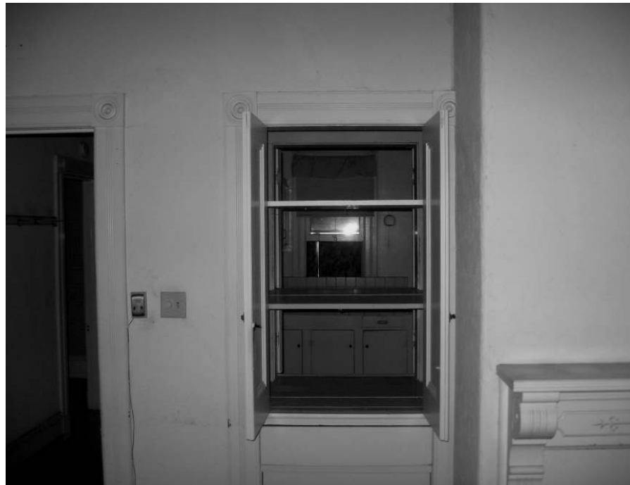
Photo 21: View of pass-through between the kitchen and dining room.
