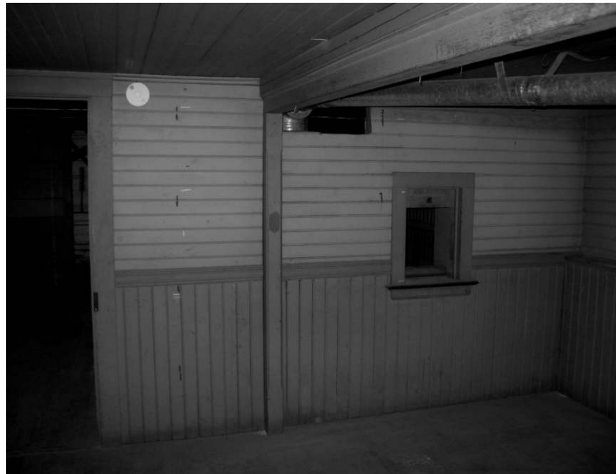
Photo 37: View of finished portion of basement with wainscoting.
