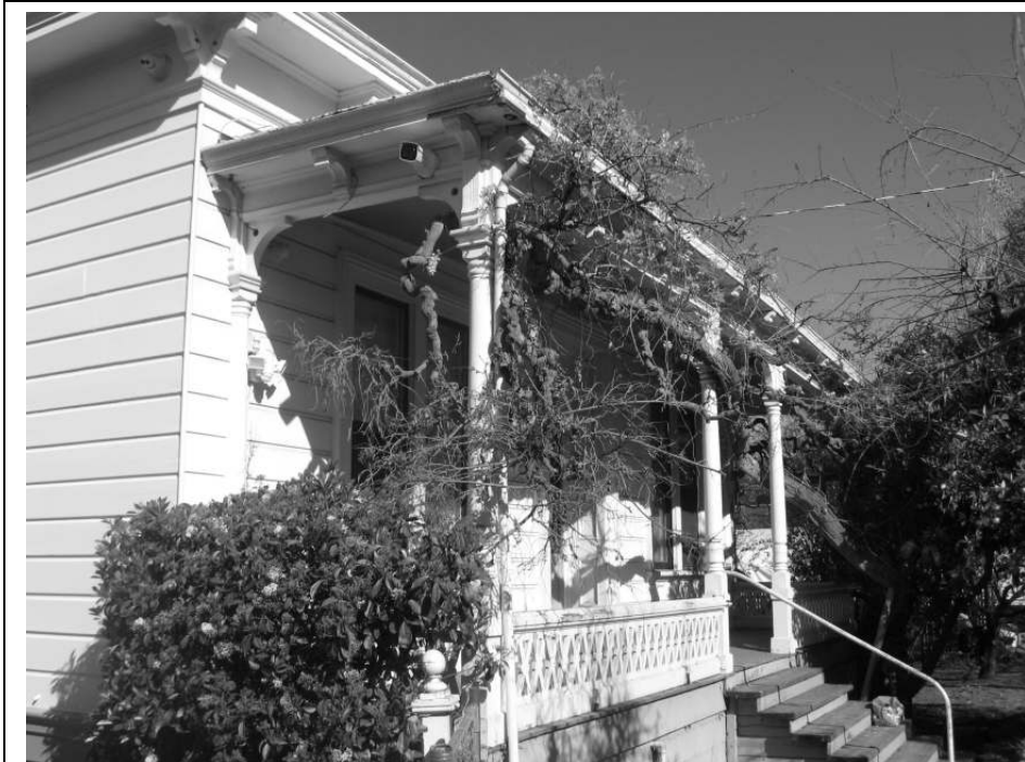
Photo 4: Oblique view of the front porch.
