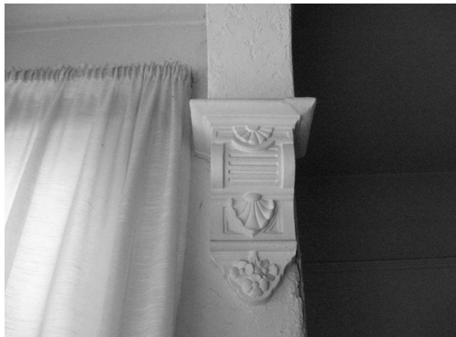
Photo 26; Detail of decorative arch support on the bay.
