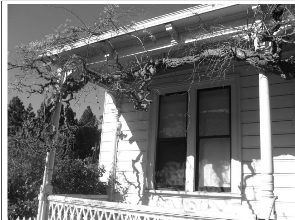
Photo 3: View of the southern portion of the front porch.
