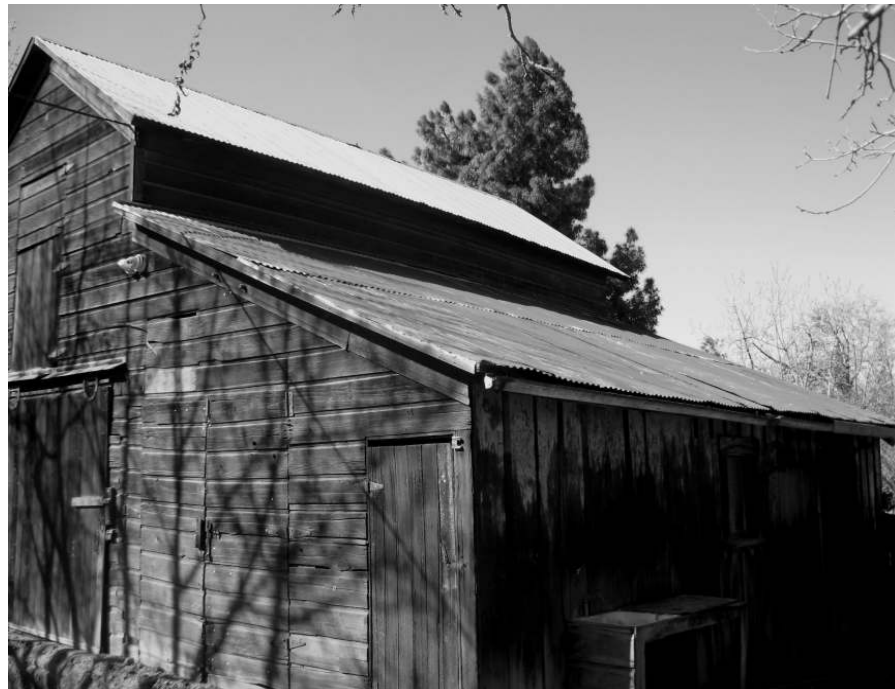
Photo 45: Oblique view of the barn from the northeast.
