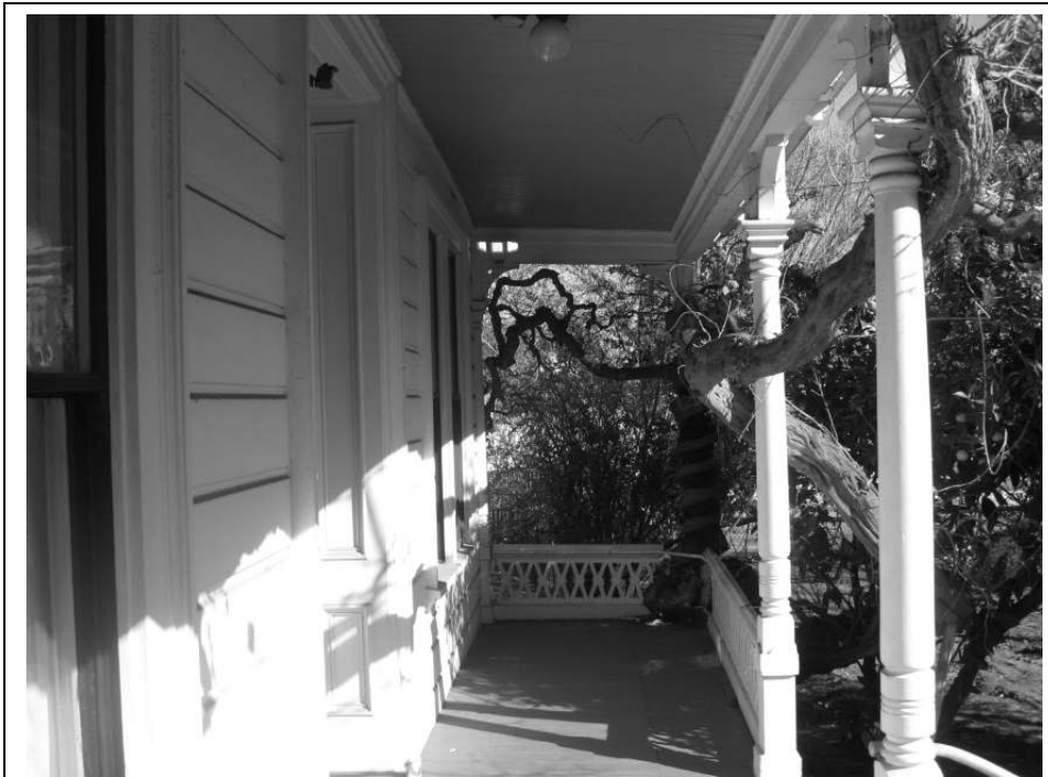
Photo 5: View along the front porch.
