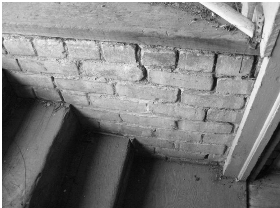
Photo 34: Detail of brick foundation in basement entry.
