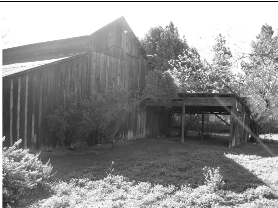
Photo 46: View of the rear facade of the barn showing shed addition.
