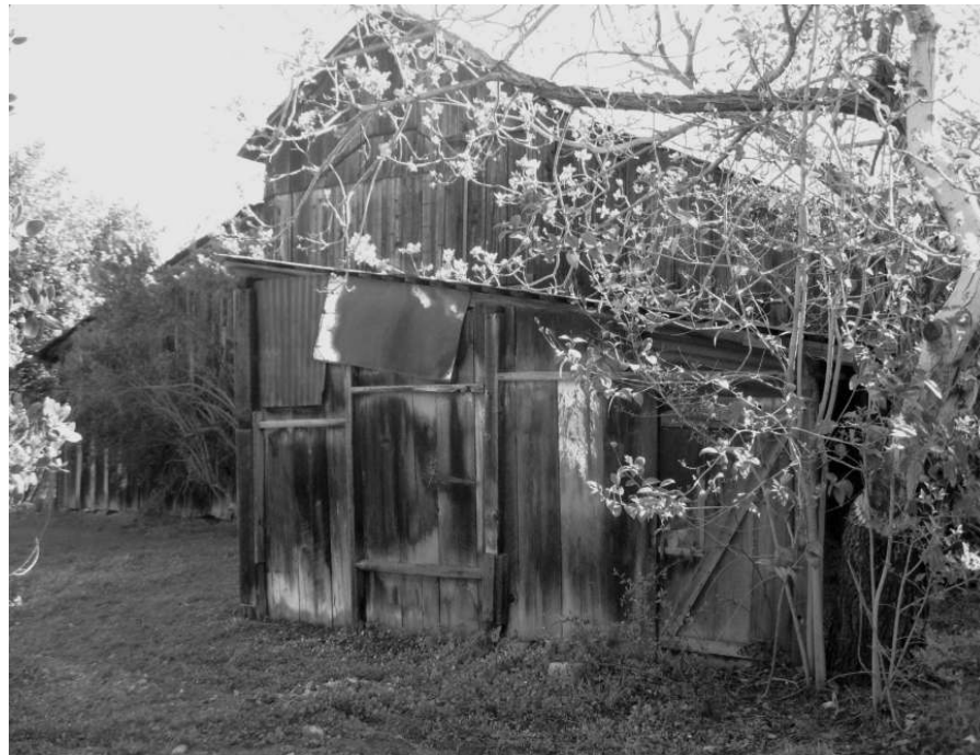
Photo 47: View of the shed roof addition to the barn.
