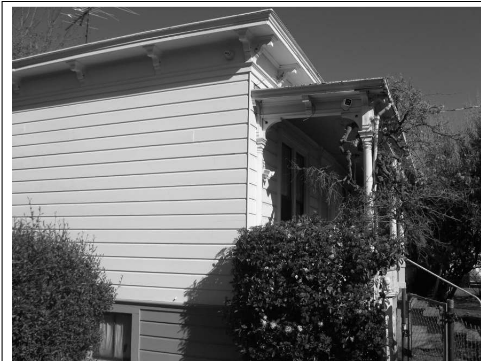
Photo 7: View of the front portion of the southern facade.
