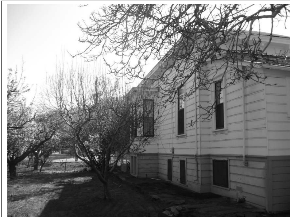
Photo 13: View along the northern facade from the northwest.
