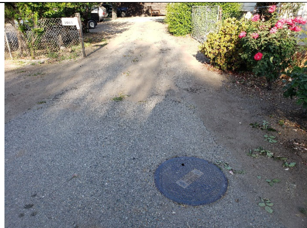
Photograph No. 5. View of city sewer system at front of property.
