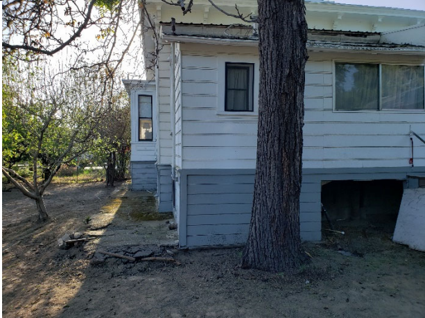
Photograph No. 13. View of northwest portion of house.
