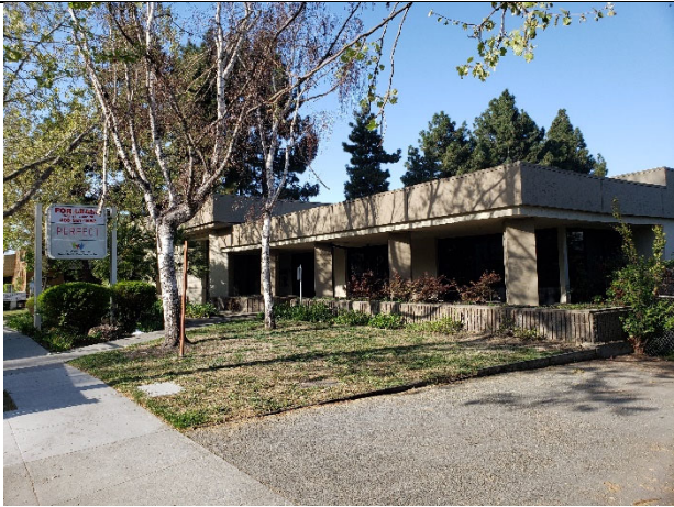
Photograph No. 27. View of commercial office building south of property.
