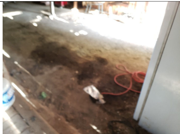
Photograph No. 23. View of oil stain on ground in barn.
