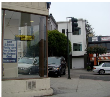
A Market Street building with a transparent corner may lead birds to think the tree is reachable by flying through the glass.
