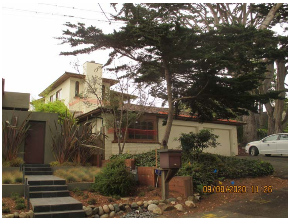
3b – Staking & flagging of proposed structure alterations.
