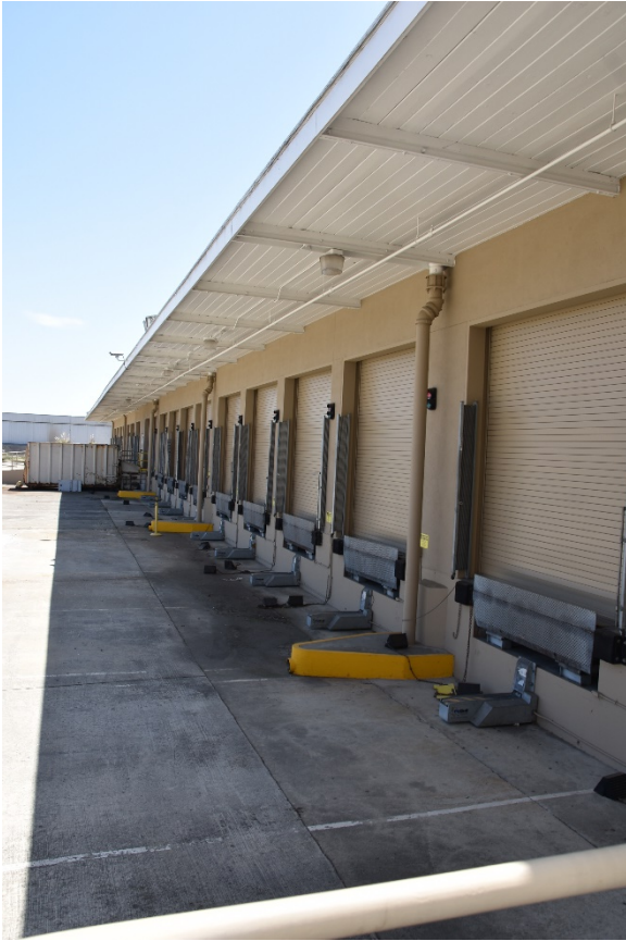
Picture 7: Warehouse loading doors at east elevation
