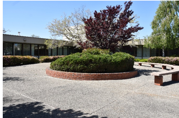
Photo 4: South elevation of east wing and east elevation of south wing from building courtyard
