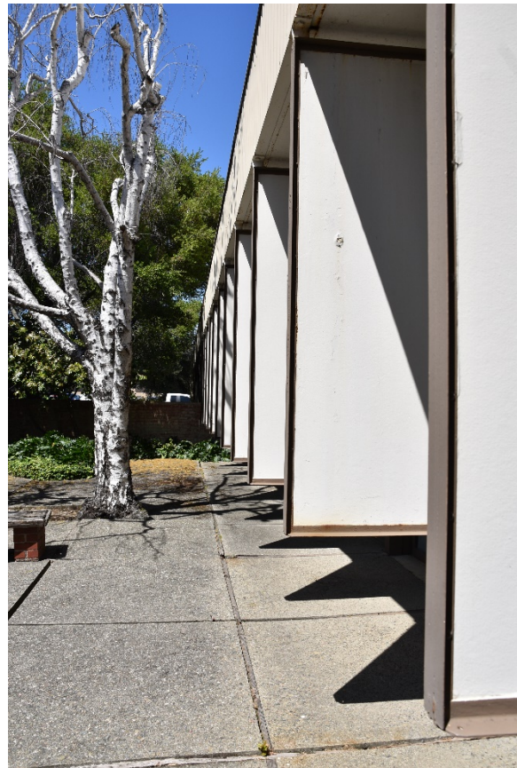
Photo 2: West elevation of fin details at the building's north wing.
