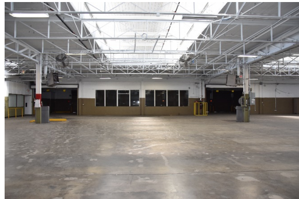
Picture 8: Warehouse interior, monitor roof above
