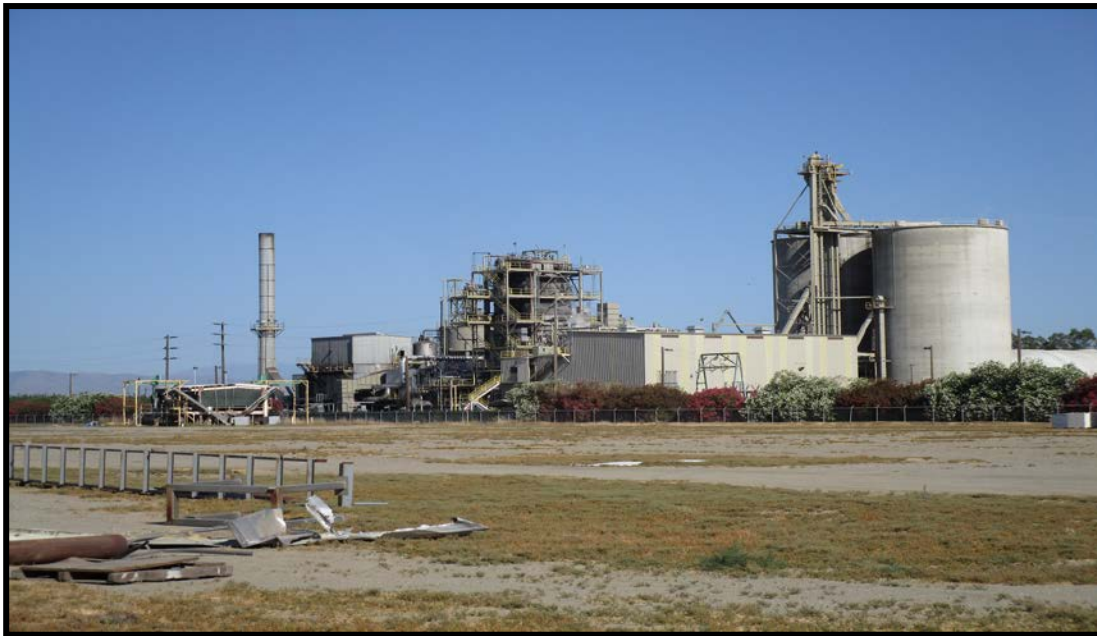
Exhibit 5 – Property to the North (Wadham Facility)
