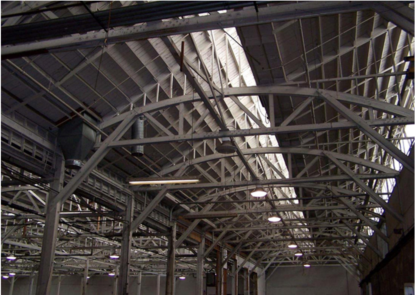
Figure 3.4-3. Former FMC Plant 1 Building A, Bowstring Truss and Sawtooth Roof Looking West/Southwest (Photo taken in 2019)
