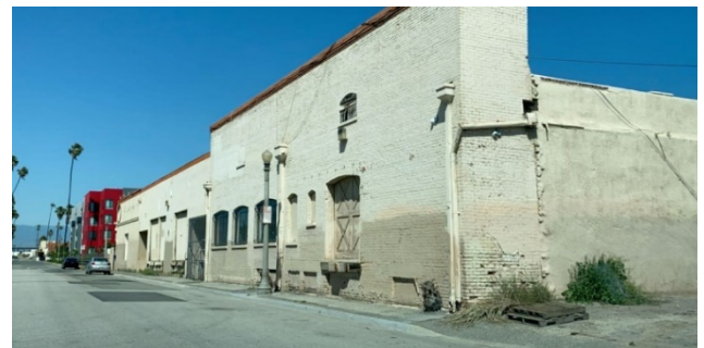
Figure 3.4-18. 3820 (foreground) and 3888 Commerce Street
