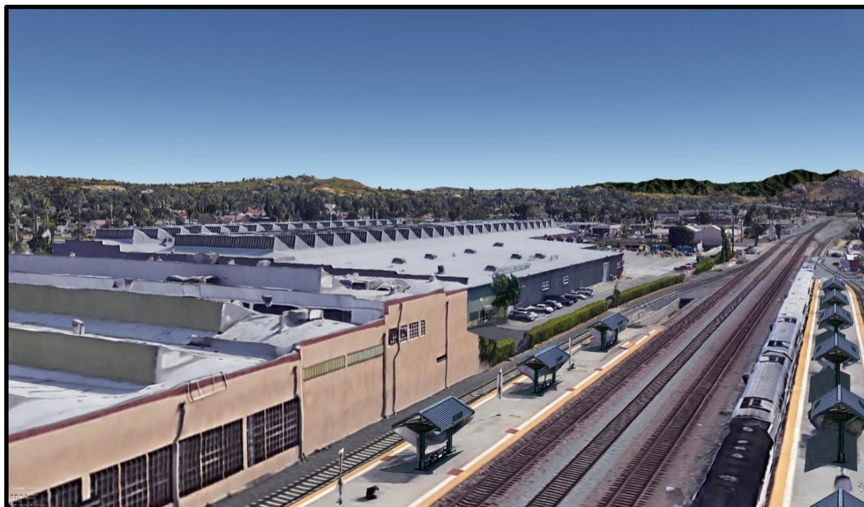
Figure 4-1. View of FMC Plants 1 and 2 and Metrolink Station, Looking Southeast (Existing)
