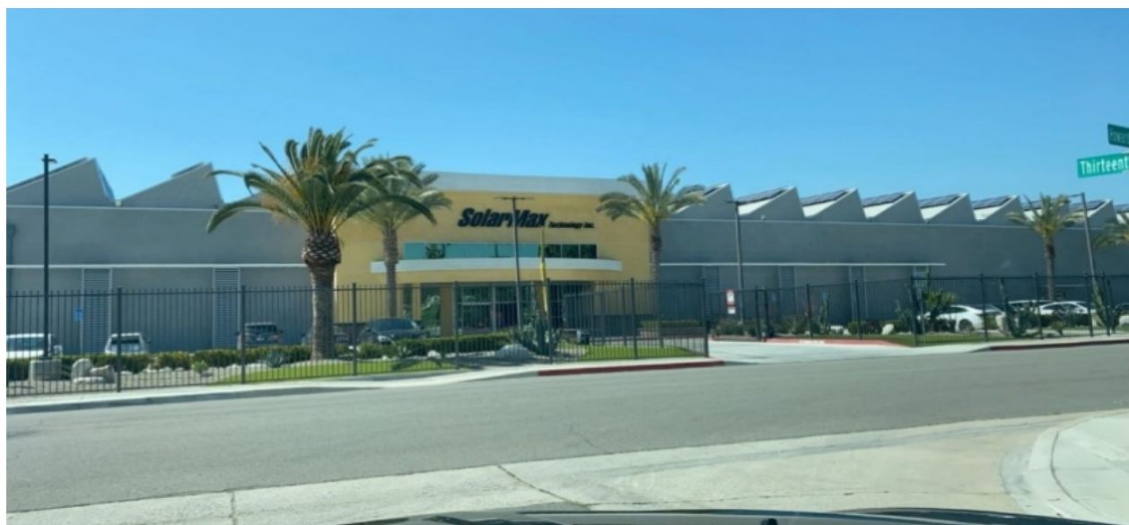
Figure 3-5. Plant 2 (Solarmax) East Elevation
