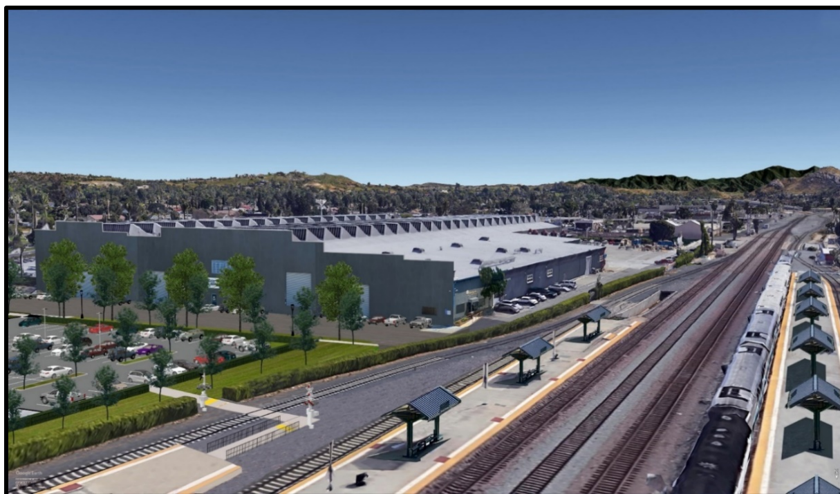
Figure 4-2. FMC Complex Plant 1 and Plant 2 with Project (Proposed)
