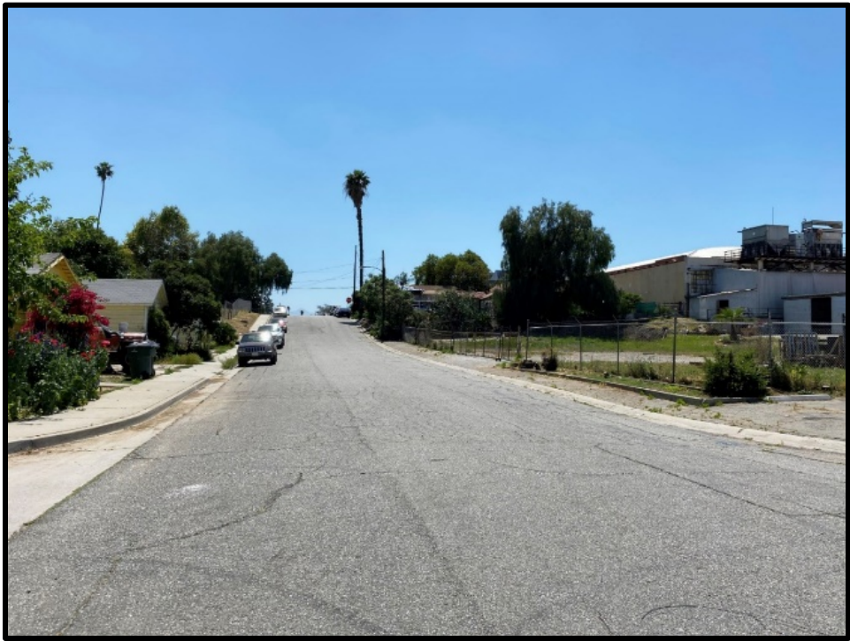
Figure 4-3. 11 th and Howard Avenue (Existing) Looking South
