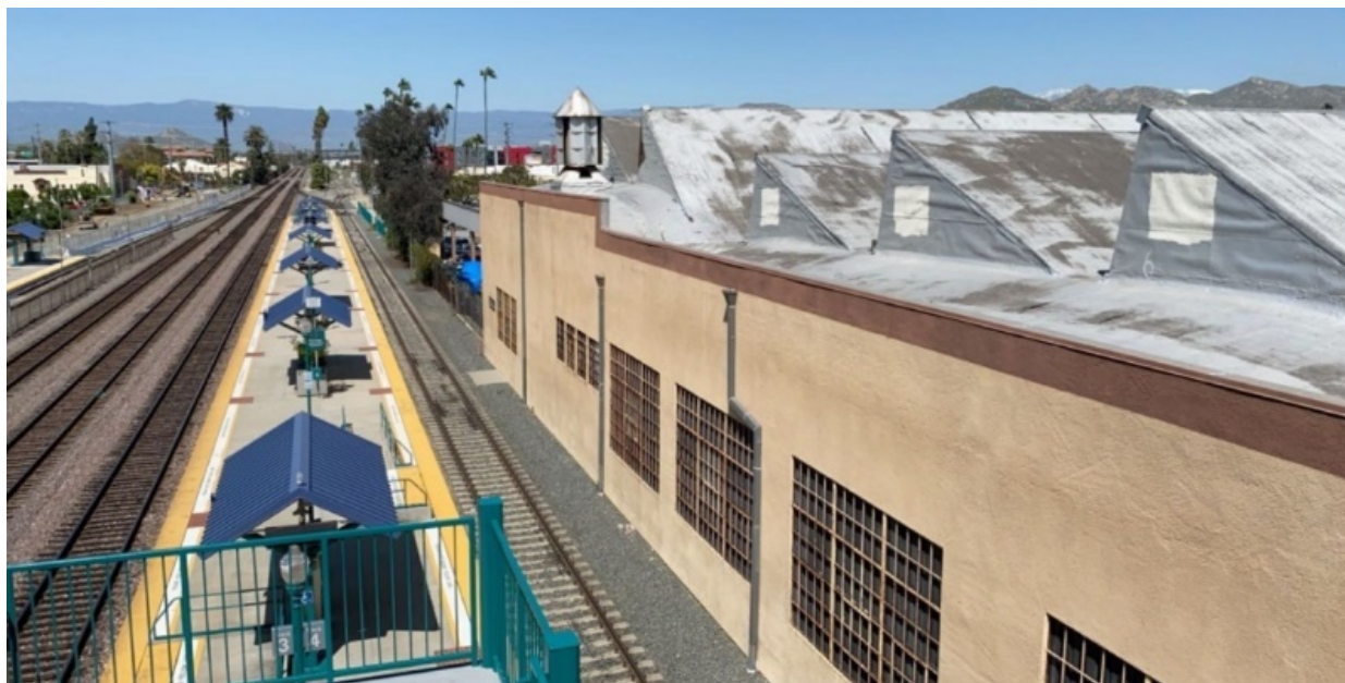
Figure 3-3. FMC Plant 1 Building A West Elevation Looking Northeast
