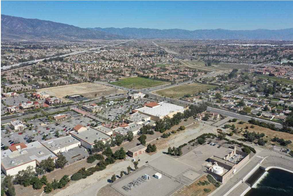
Figure 3i Aerial View towards Project Site Facing Northeast
