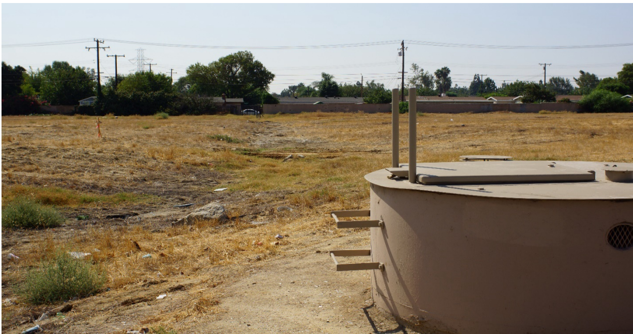
Plate 2: Unlined storm drain channel and vault, view south.
