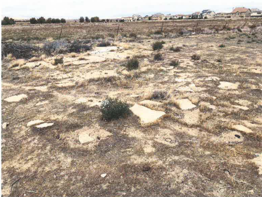
Photo 4: Feature 5, foundation, view northwest.
