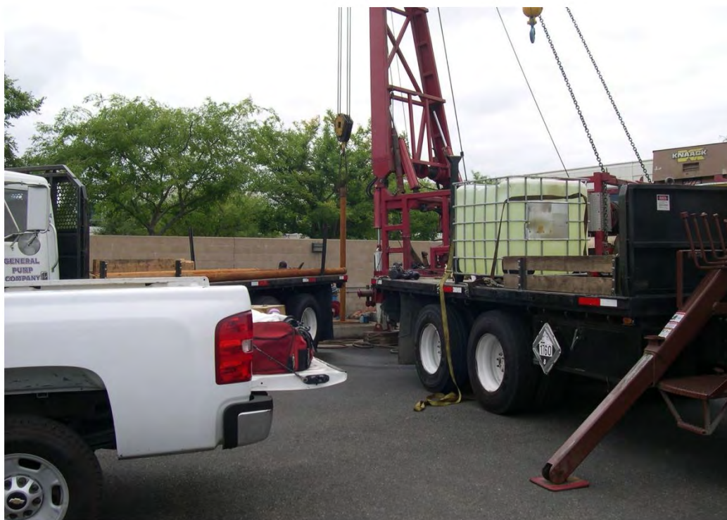
Photo 2: Well Rehabilitation Activities
