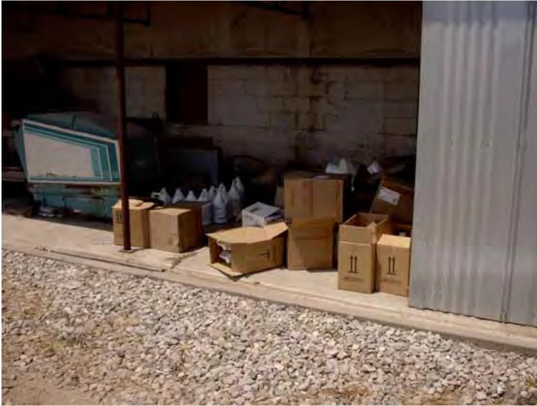
View of several chemicals stored outside at the chemical storage building.
