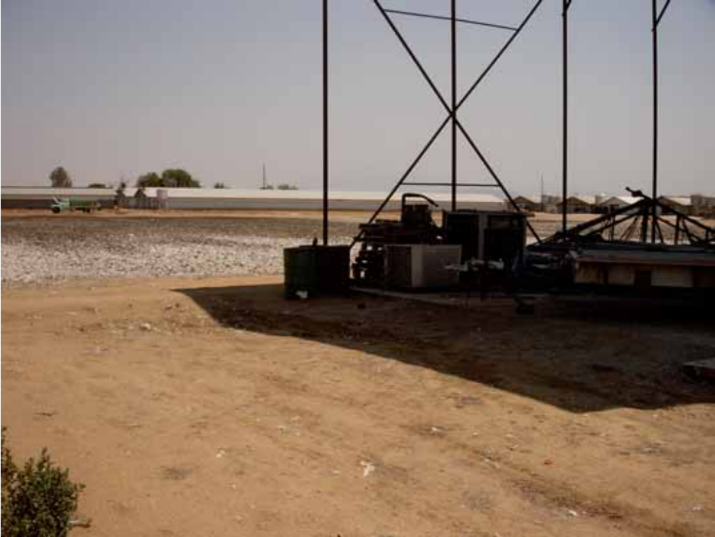
Looking east at various equipment and drums in structure without siding.
