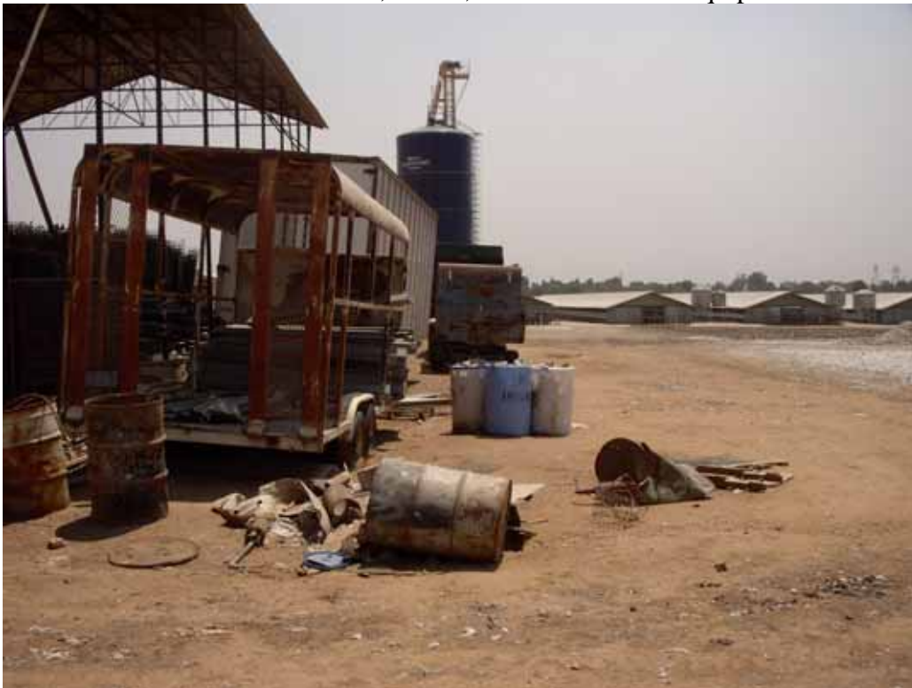
Looking south at drums and other trash near structure without siding.
