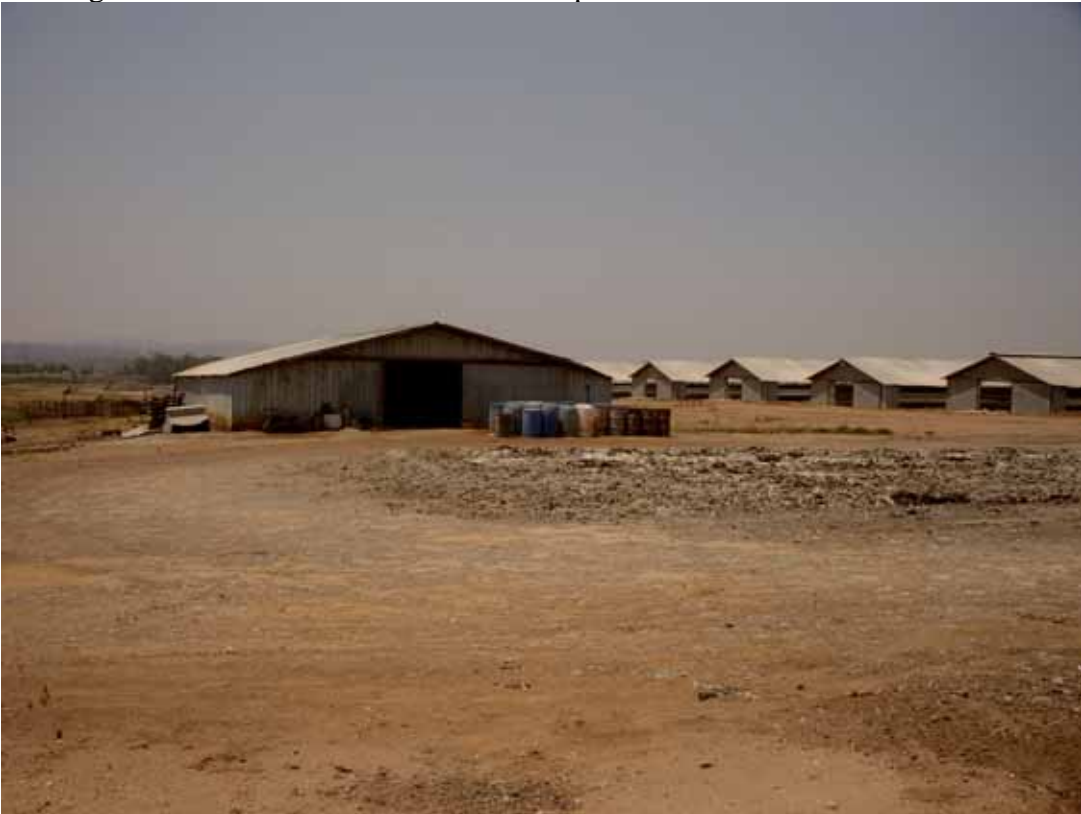
View to west of pig barn, south site boundary to the left of photo and chicken coops to the right side of photo and spread manure in foreground.
