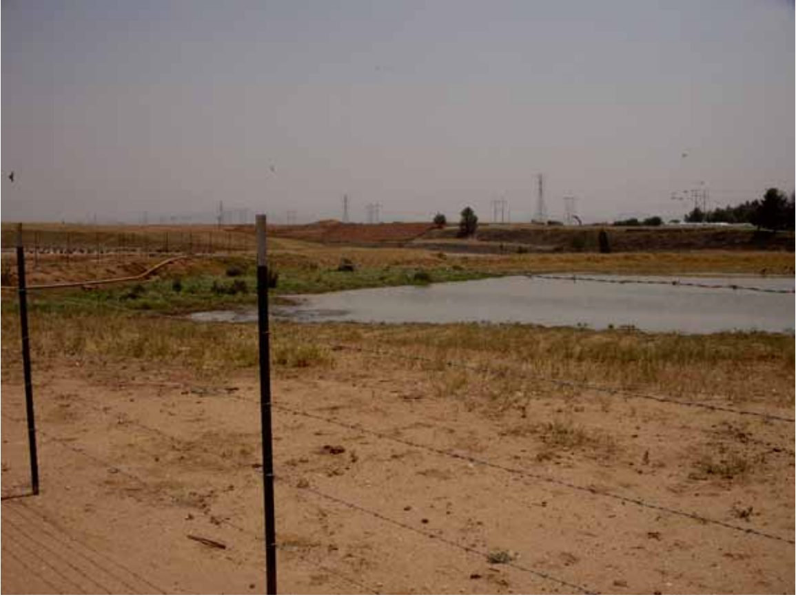
View to southeast of southeastern most retention pond.
