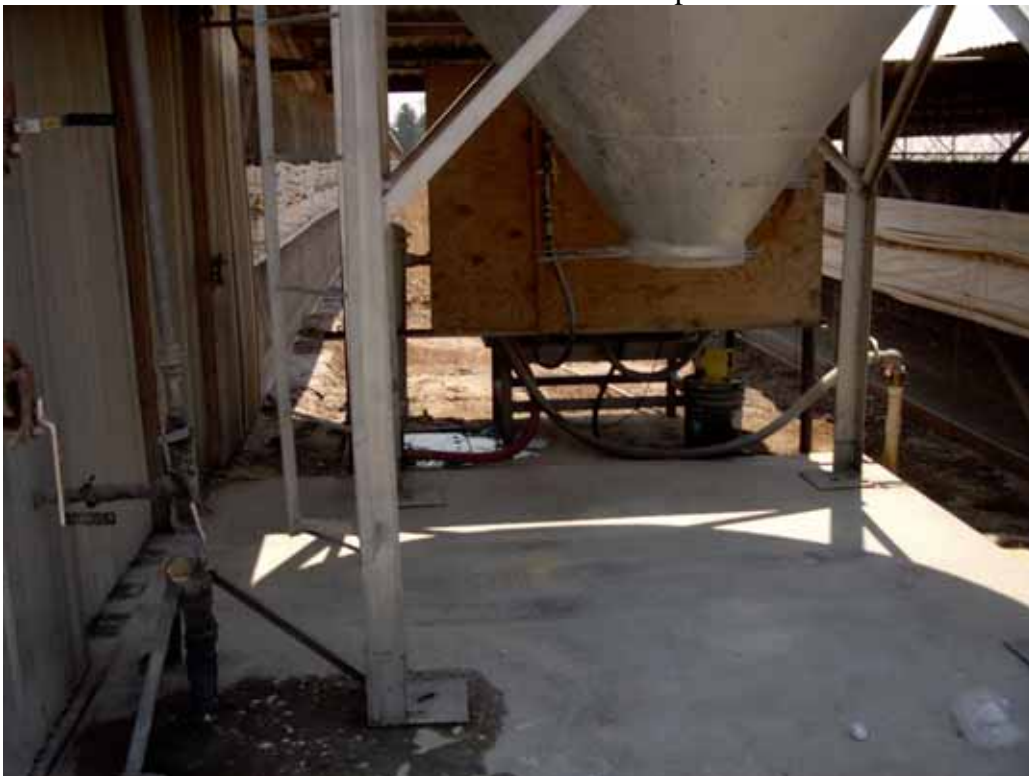
Picture of water leaking onto ground surface from ranching equipment.
