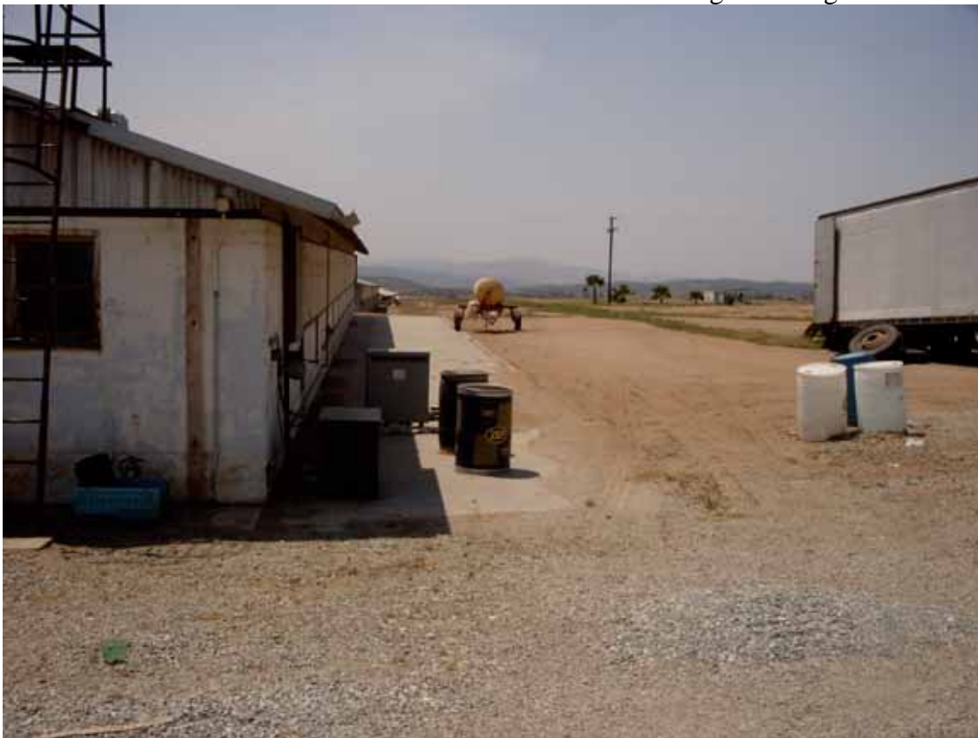
View to west of north side of chemical storage building and various drums and tanks.
