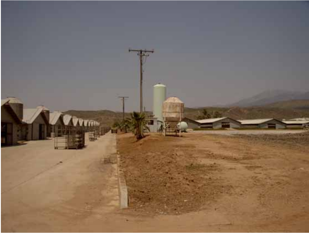
Green water tank for holding groundwater at one of the site production wells.
