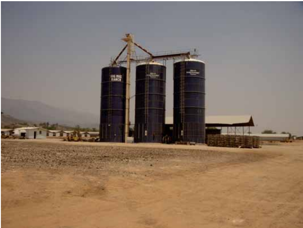
Three silos shown with bathroom to the left and misc. farm equipment.
