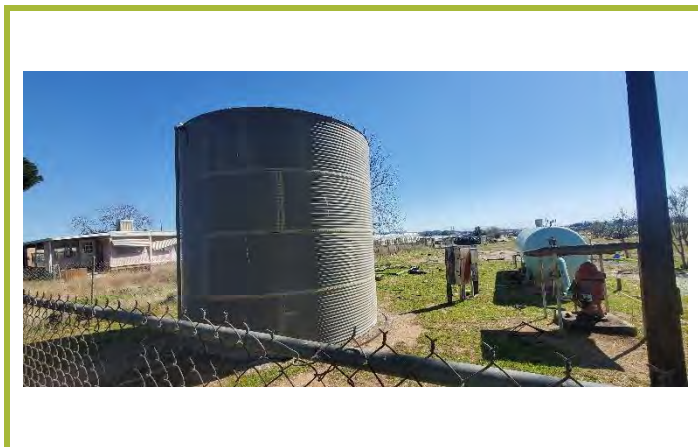
Photograph #8: View of an AST on the northeast portion of the site.
