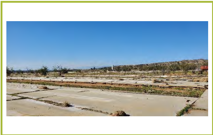
Photograph #2: Additional overview of the site.
