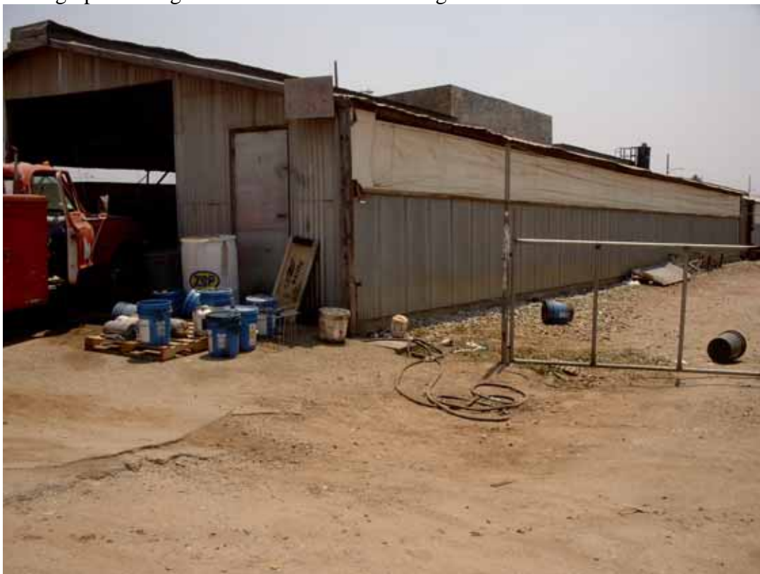
Photograph looking south at building housing diesel power backup equipment.
