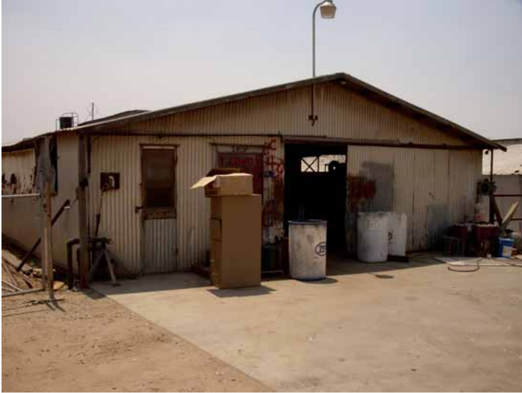
Photograph looking south at mechanical building.
