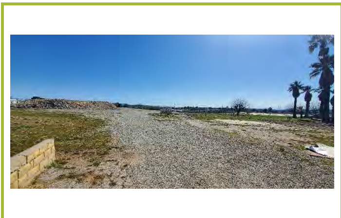
Photograph #7: View of a demolished agricultural building (left) and abandoned agricultural building (right).
