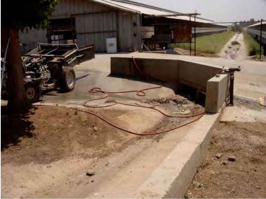
Washout area to the southwest of the silos.
