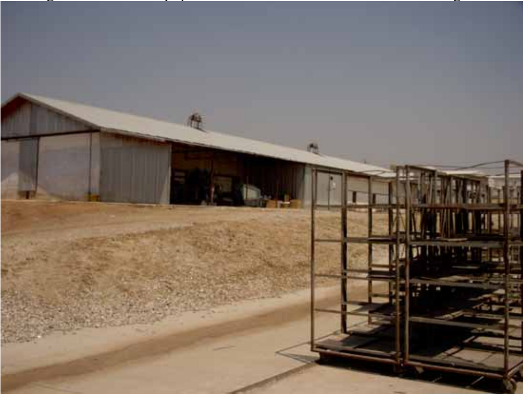
Looking northeast at pesticide and chemical storage building.
