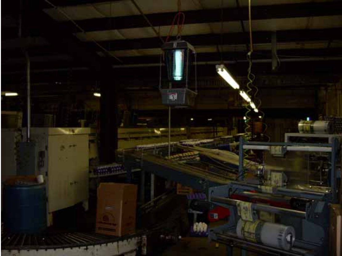
Processing plant area looking east inside building.
