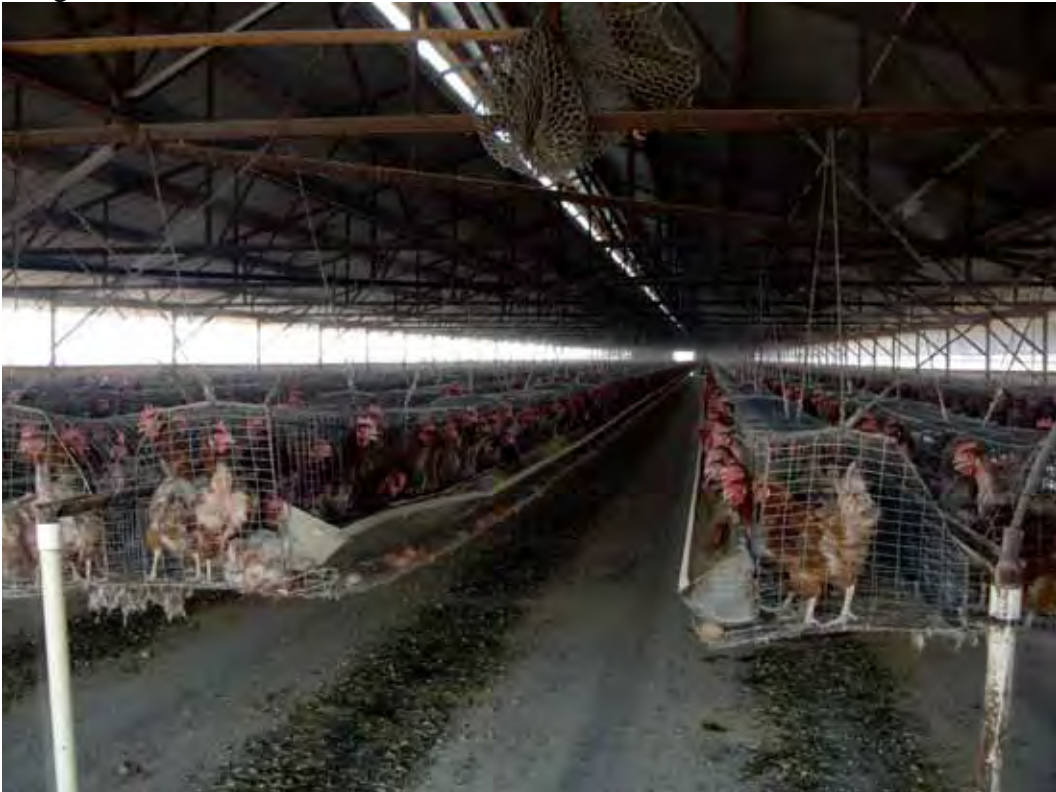
View inside chicken coop showing concrete slab on grade and suspended coops.
