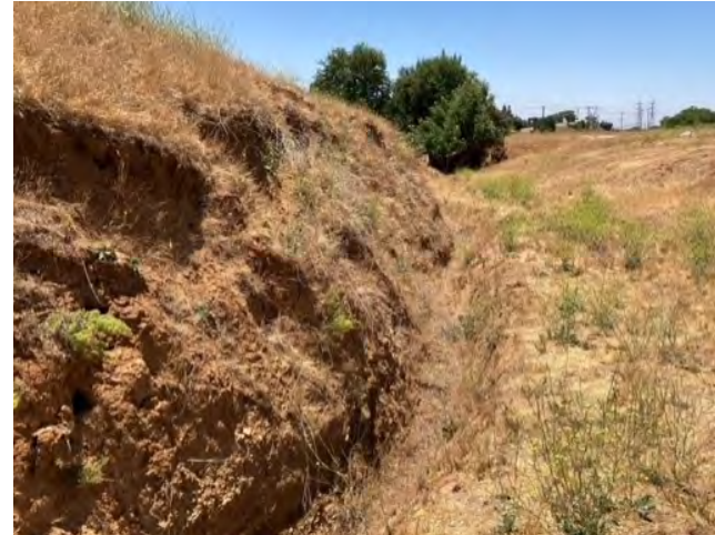
Photo 30. Downstream view of NWW-3A, facing southwest (33.962811, -117.018492). June 3, 2021.
