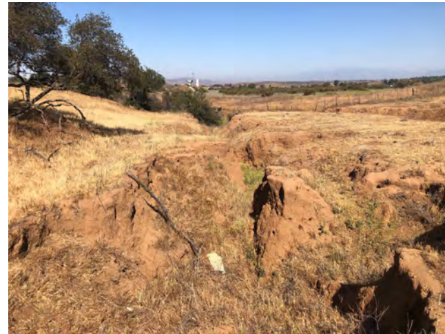
Photo 10. Downstream view of NWW-1 from upstream extent, facing west. As NWW-1 continues downstream, OHWM indicators become more prominent (33.965835, -117.024734). June 3, 2021.
