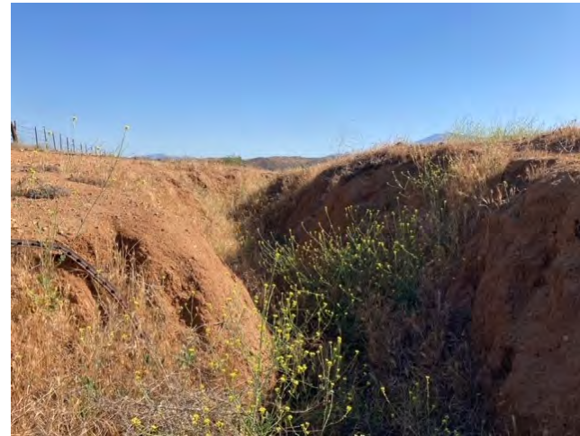
Photo 4. View of ODP 2, facing southwest, within EF-2. The gully/erosional feature exhibited a slight break in bank slope but did not exhibit a distinctive change in average sediment texture, change in vegetation species or cover, or any other OHWM indicators, and did not continue downstream (33.967305, -117.025013). June 3, 2021.
