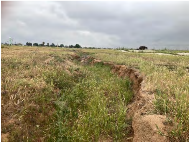
Photo 39. View of D-1, facing east (33.965103, -117.019365). April 22, 2021.
