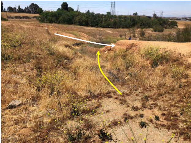
Photo 37. View of EF-7 (yellow arrow), just south of EF-6, facing south/southwest. EF-7 converges with EF-8 (white arrow), neither of which appeared to contribute flows to NWW-3B (33.963581, -117.020494). June 3, 2021.
