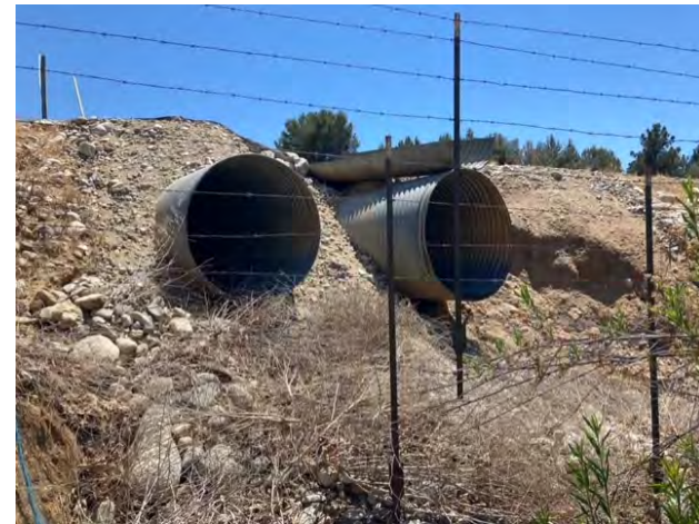
Photo 22. View of culvert outlets located along the southern extent of the review area under Brookside Avenue, facing south. Flows from the culvert outlets continue into NWW-3 (33.961603, -117.018517). June 3, 2021.
