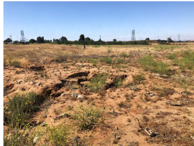
Photo 40. View of area where D-1 abruptly stops, facing south. Flows likely continue as sheet flow into S-5, before continuing into NWW-3B1 (33.964824, -117.020845). June 3, 2021.
