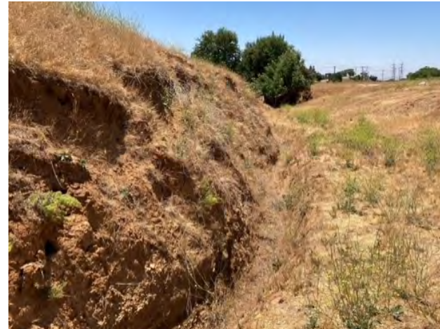
Photo 30. Downstream view of NWW-3A, facing southwest (33.962811, -117.018492). June 3, 2021.
