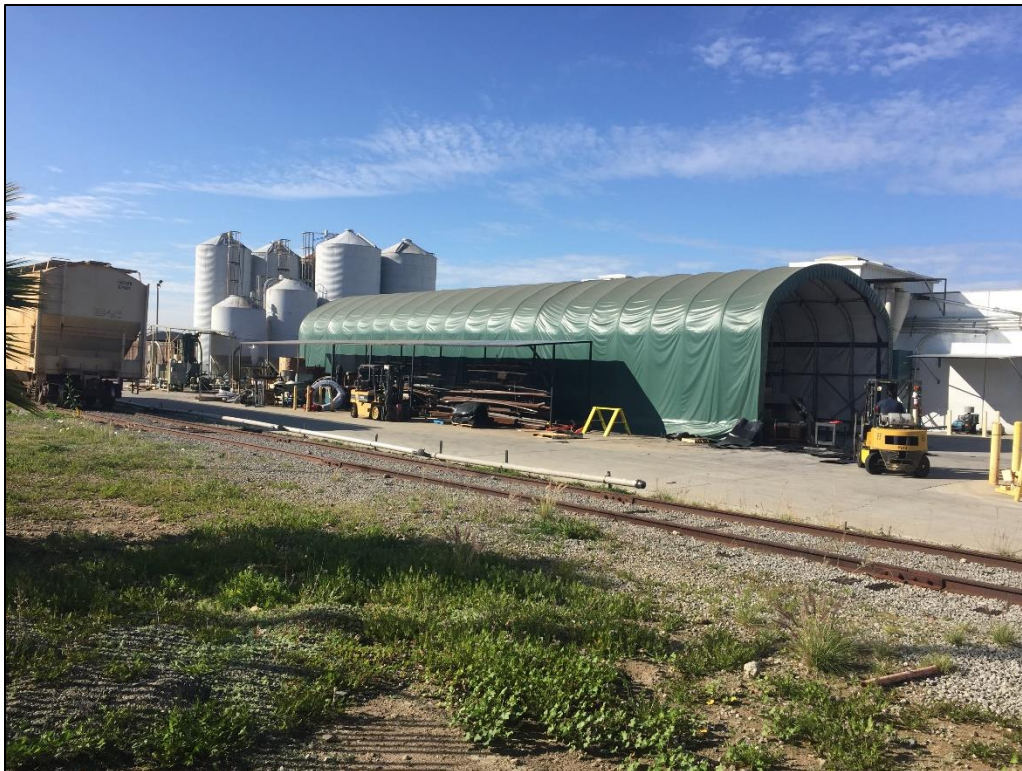
Figure 3. View of BNSF Railroad spur, warehouse building, and silos from within Project near northeast corner of Project. View to southwest.
