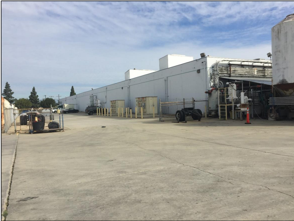
Figure 4. Southwest corner of existing building. View northeast.
