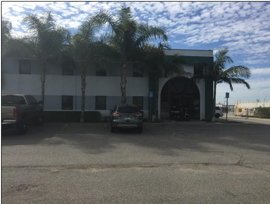
Figure 1. View of north side of existing warehouse building, to be demolished. View south.
