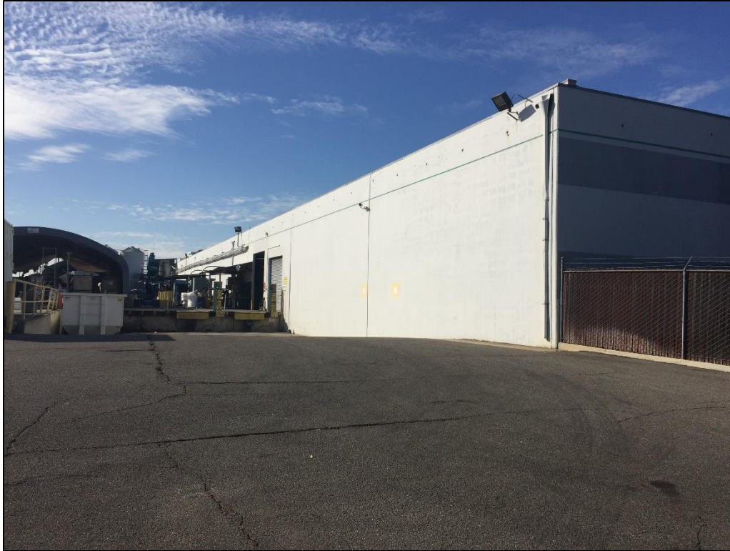
Figure 2. Northeast corner of existing building. View south-southwest.
