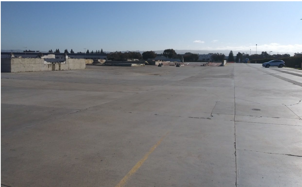
Photograph 4. Paved areas of the site
