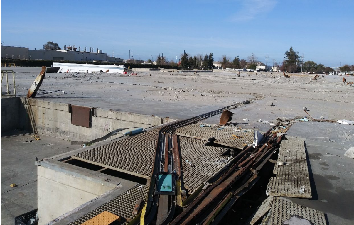
Photograph 3. Remaining Berkeley Farms foundation
