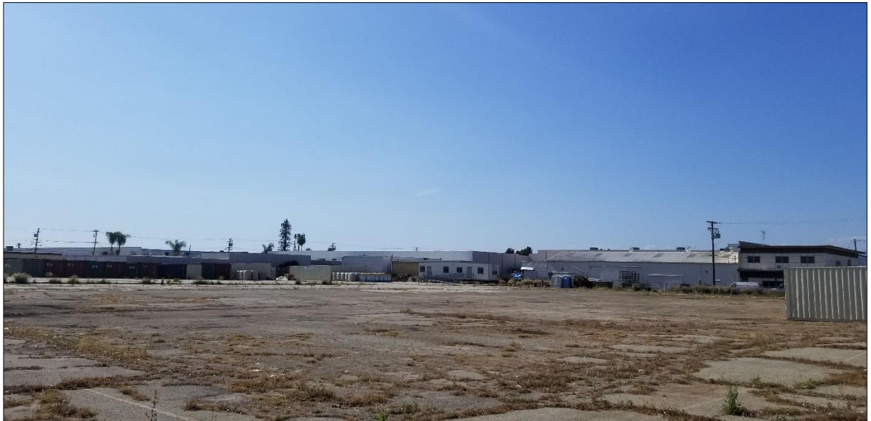
Figure 2: The larger 3.93-acre site of the development (Area 1) would include a two 2-story courtyard style wood-frame walk up buildings, and one 3-story wood-frame building with an elevator and interior corridor. This portion of the multiple-family housing complex west of Laurel Avenue would include 121 residential units, along with staff offices and resident amenities.
