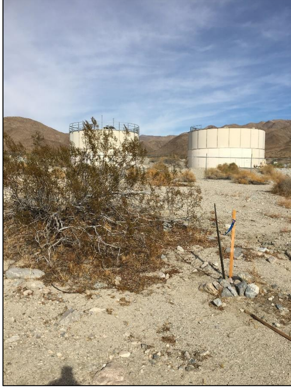
Photograph 3: Project survey boundary SW corner, Transect 2, facing North
