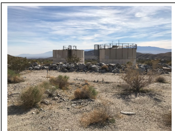
The Project site is located in a generally flat to gently sloping desert landscape near the base of the Little San Bernardino Mountains to the north and east and distant mountain views to the south and west. The Project site has been previously disturbed and developed with two 35-foot diameter, 16-foot-tall bolted-steel tanks.
