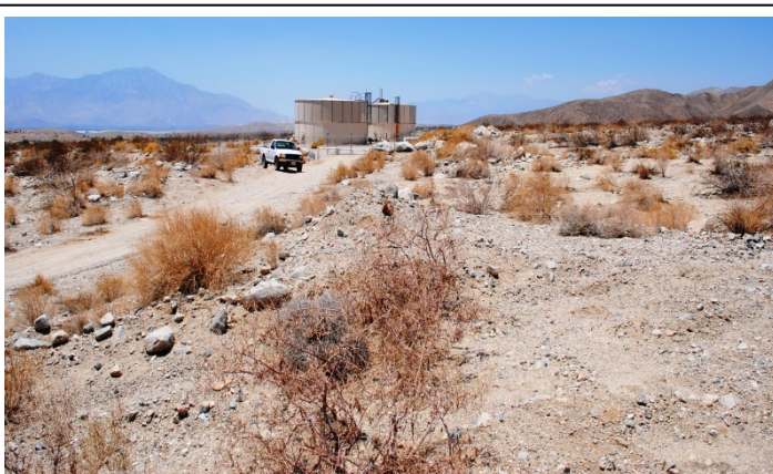
The Project site is currently developed with existing Reservoirs 4711-1 and 4711-2. These tanks would be demolished following construction and initial operation of the proposed 1MG Reservoirs 4711-3 and 4711-4.
