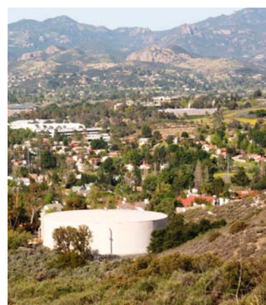
Las Virgenes Municipal Water District storage tank
