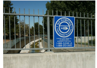
Flood control and storm water facilities
