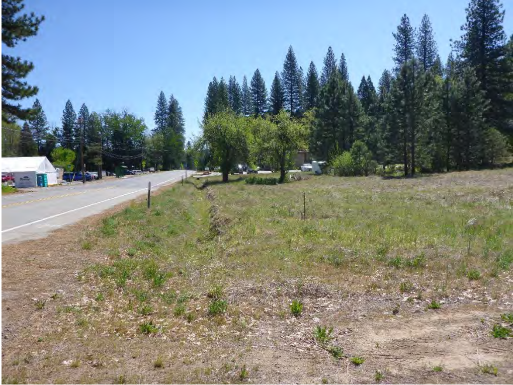
Roadside ditch parallel to Bucks Lake Road with site access road in foreground, view to east
