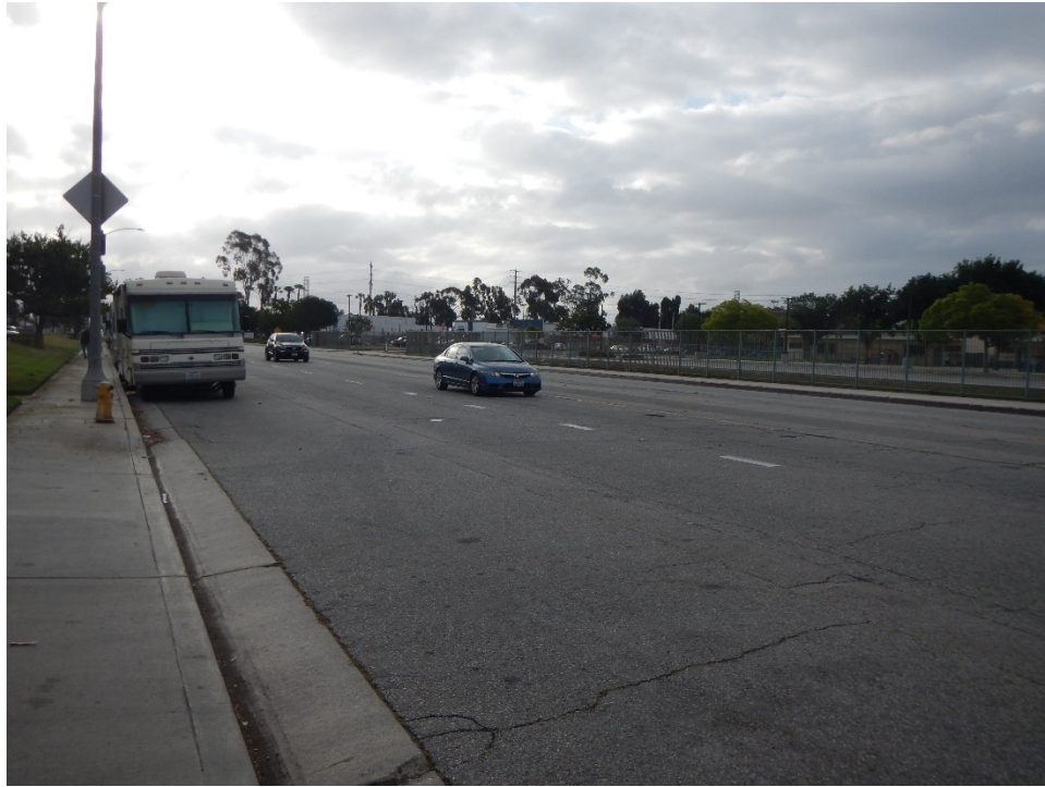
Photograph 9 – Facing east on the northern pedestrian sidewalk along Victoria Street. Water conveyance pipelines are proposed within the right-of-way.
