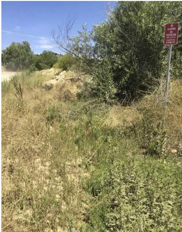
20. View of stormwater detention swale between 13th street road and Basin 1. This receives water from the paved 13th street to the south.
