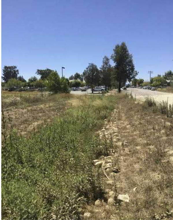
19. View of stormwater detention swale between 13th street road and Basin 1. This receives water from the paved 13th street to the south.
