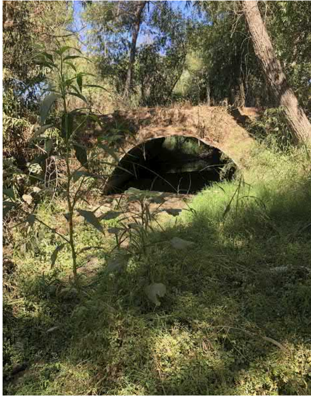
99. View of culvert outlet in Santa Maria Creek.
