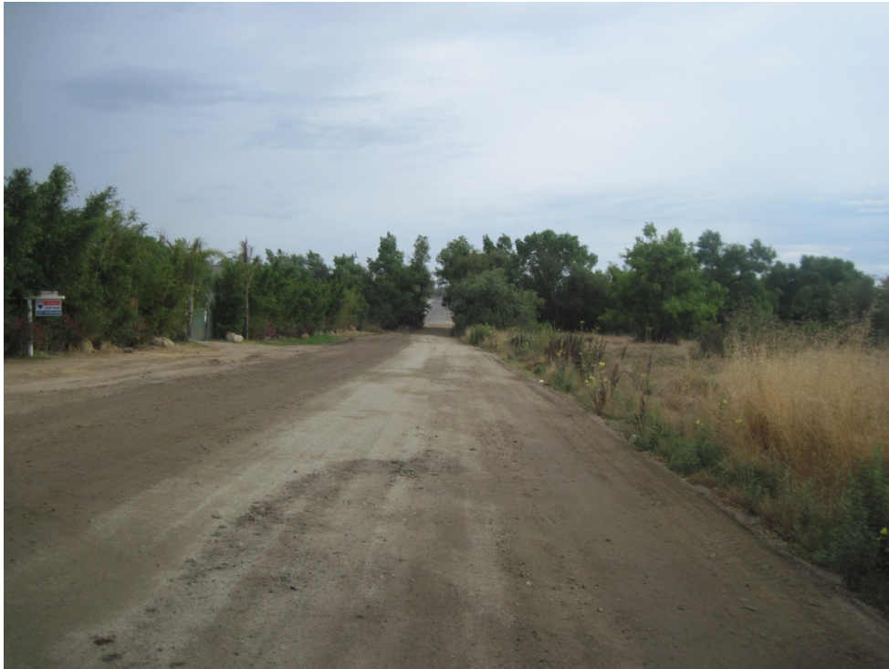
Photo 5 – View of 13 th Street, facing north.
