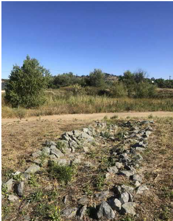
44. View of riprap stormdrain channel from the Ramona Library parking lot to Basin 1.
