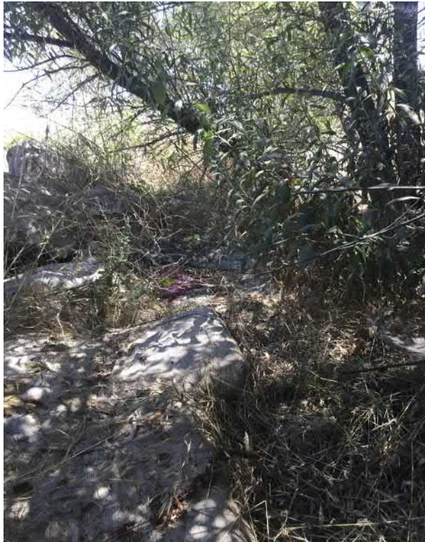
22. View of stormwater detention basin where the water from Basin 1 drains. Debris surrounding basin.
