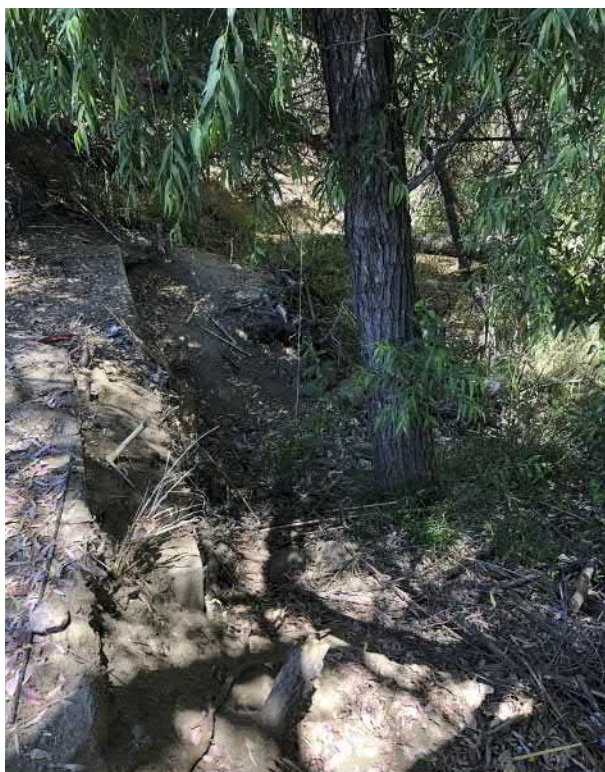
80. View of culvert outlet in Santa Maria Creek.
