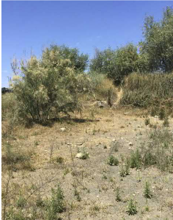
27. View of culvert in Basin 1 taken from within Basin 1.
