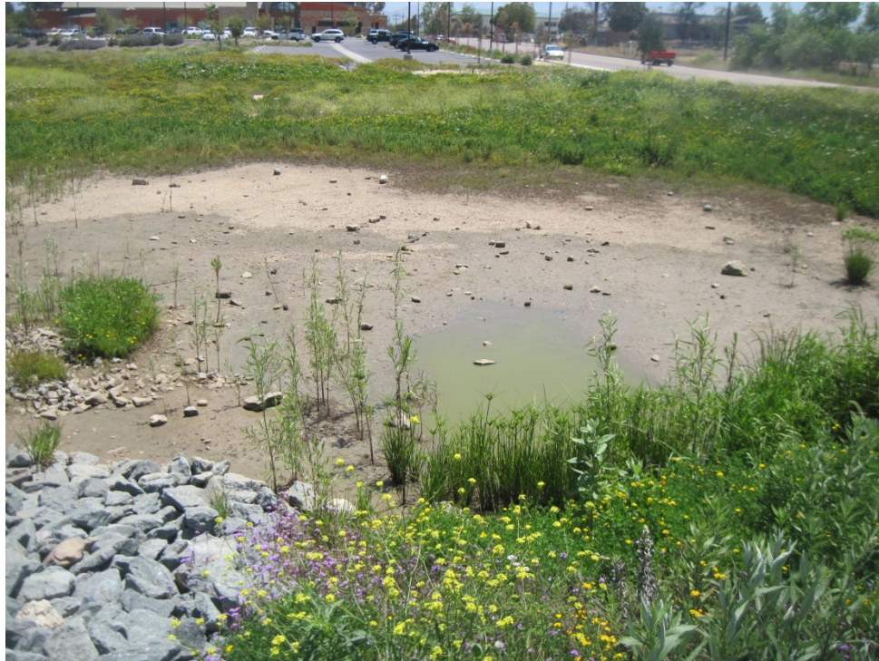
Photo 7 – View of the settling basin adjacent to the library parking lot, facing south.
