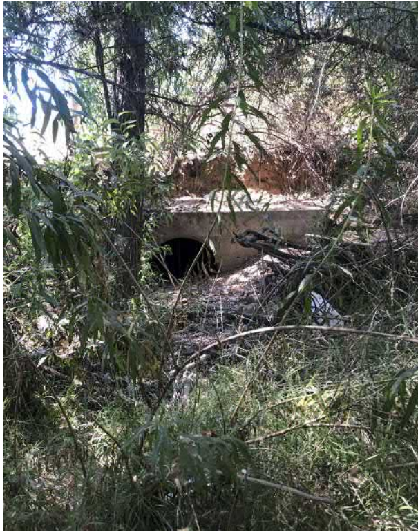
91. View of culvert outlet in Santa Maria Creek.
