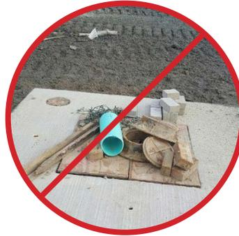
2. Final paving must be completed. Final paving ensures that paving materials will not enter and contaminate the Filterra system during the paving process, and that the plant will receive runoff from the drainage area, assisting with plant survival for the Filterra system.
