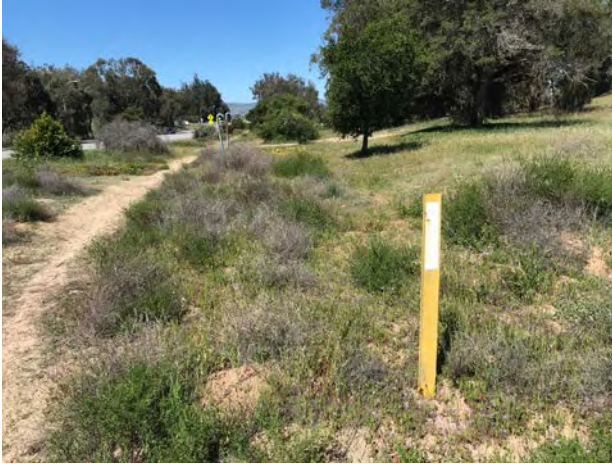
Photograph 7. View of a gas pipeline marker located along the southern boundary of the subject property, facing west.
