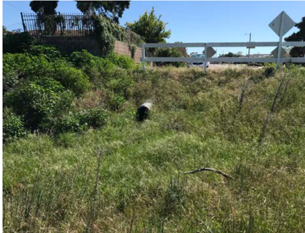
Photograph 2. View of a culvert that drains onto the subject property located along the eastern boundary, facing east.
