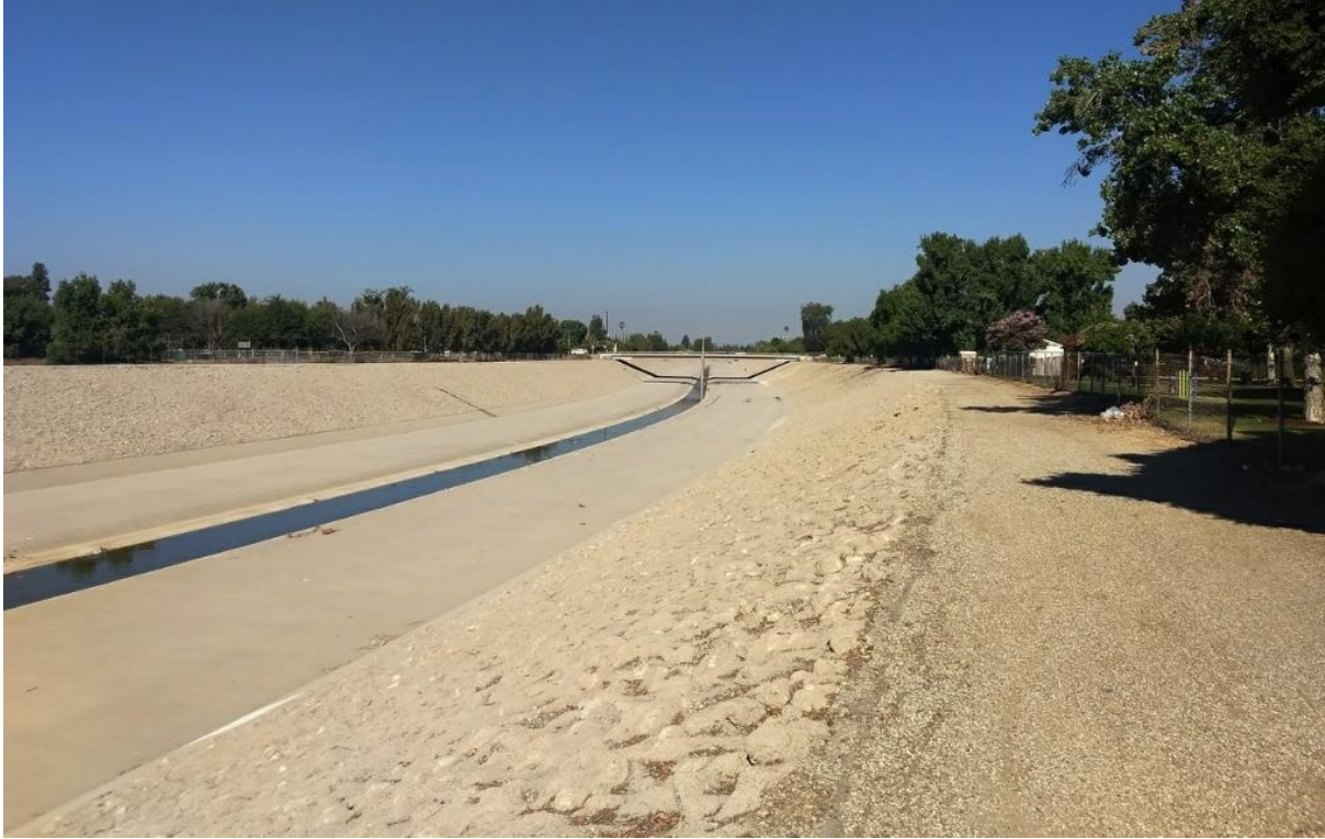
Photograph 3. Overview of concrete lined portion of Study Area east of Reseda Park. Photo facing east.
