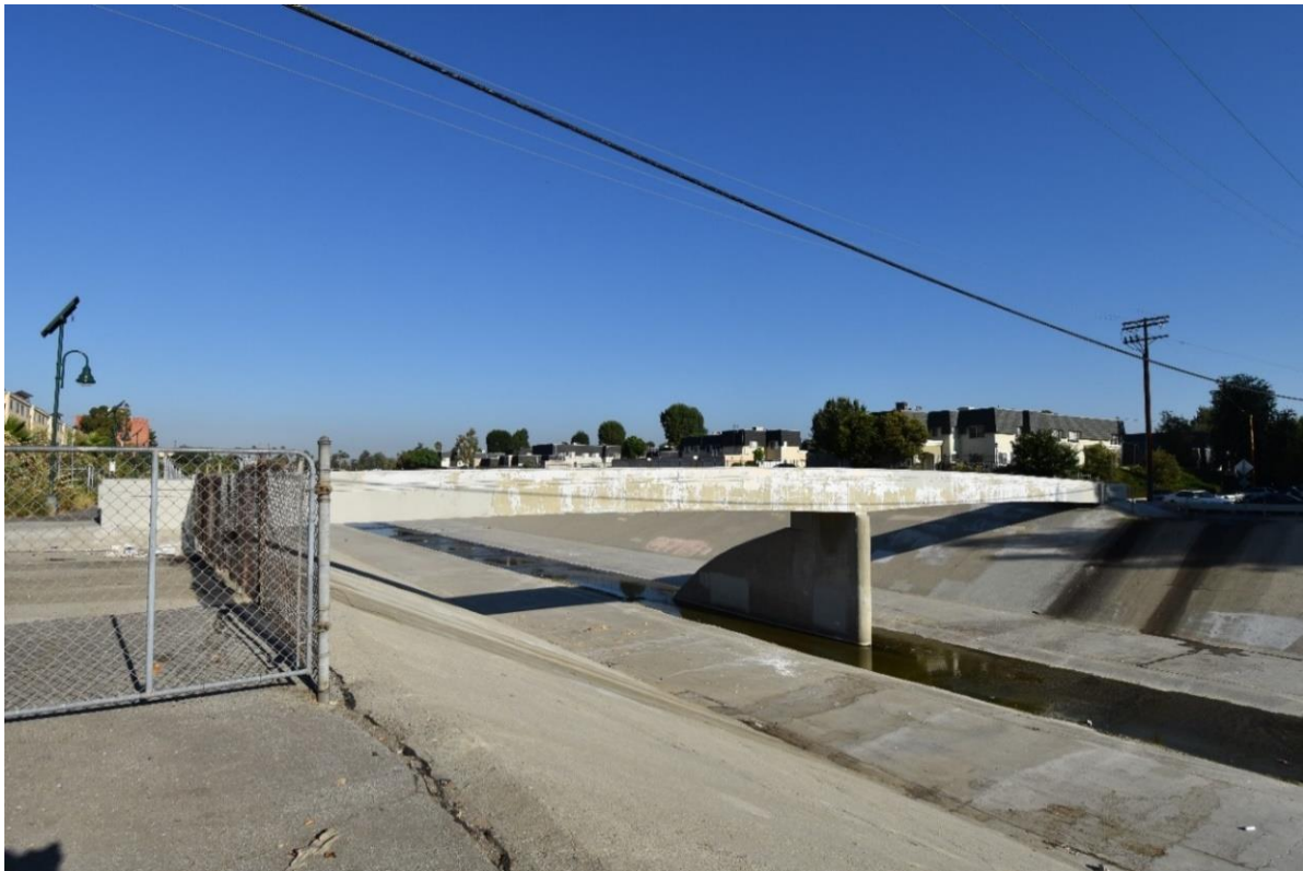
Figure 9 Vanalden Avenue Pedestrian Bridge; Photograph Taken from the Southeast, Northwest-Facing
