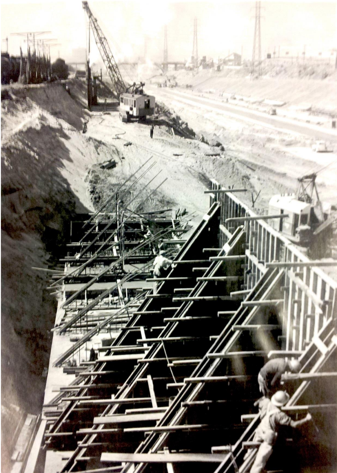
Figure 5 Construction of River Channel South of Olympic Boulevard in Los Angeles, 1939
