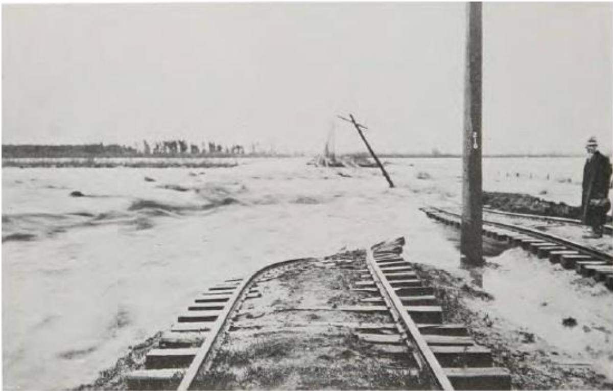
Photograph obtained from A History of the Los Angeles District-U.S. Army Corps of Engineers 1898-1965 by Anthony F. Turhollow
