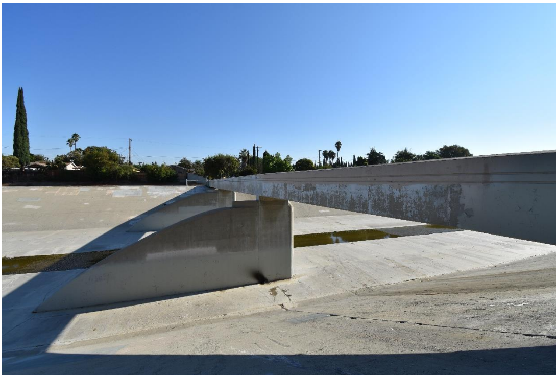
Figure 10 Amigo Avenue Pedestrian Bridge; Photograph Taken from the Southwest, Northeast-Facing
