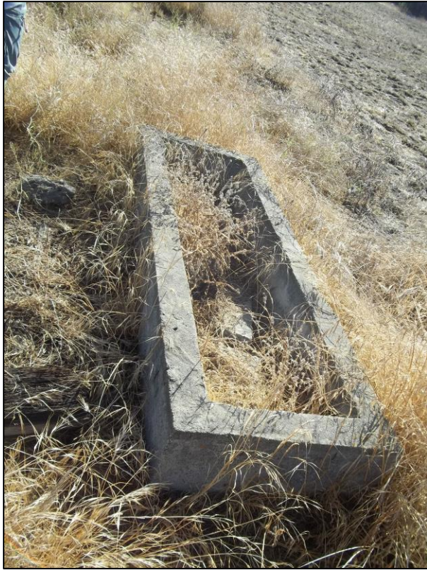
Overview of 1 of 5 concrete trough
