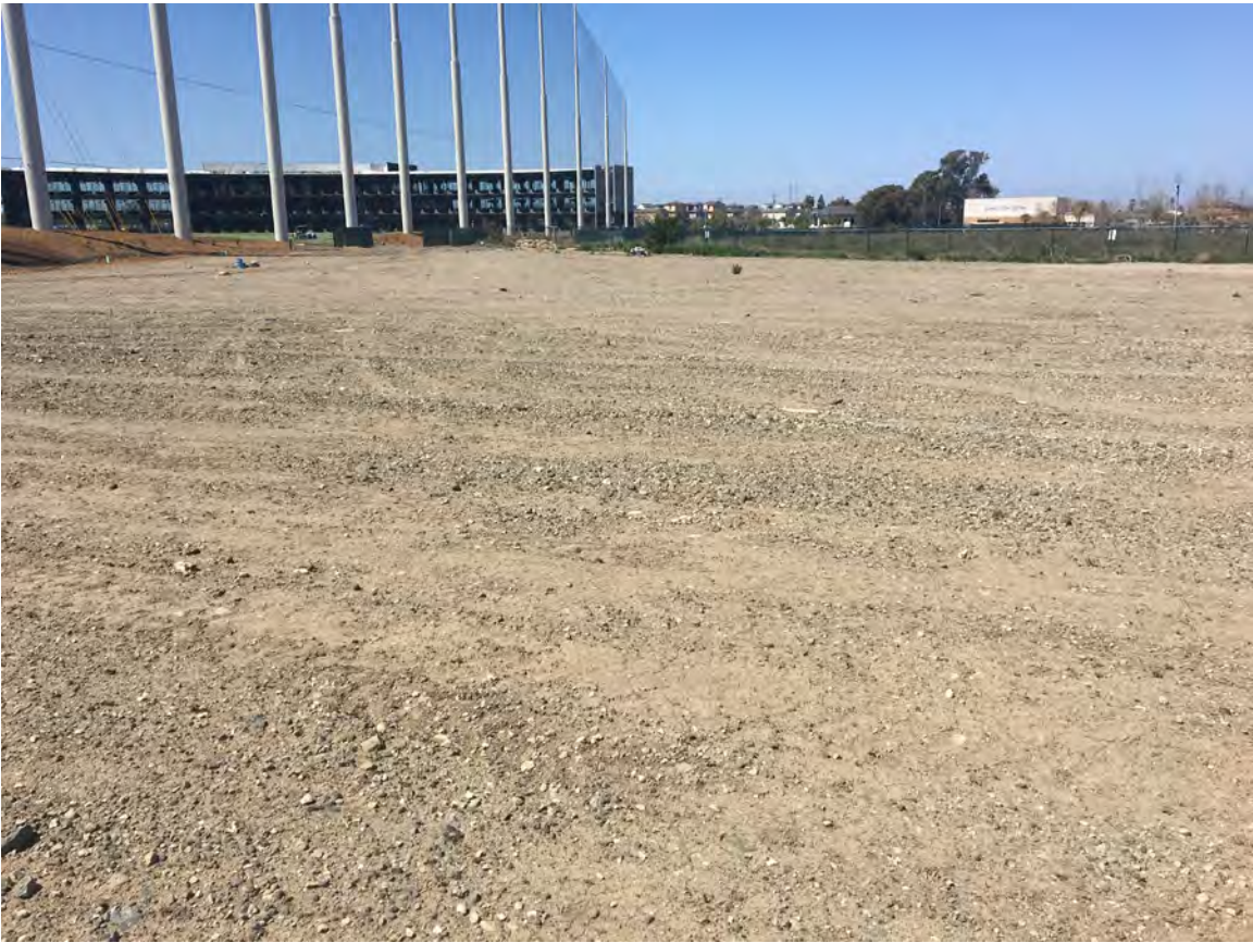
Photograph 1 - Graded area view northwest toward entrance road
