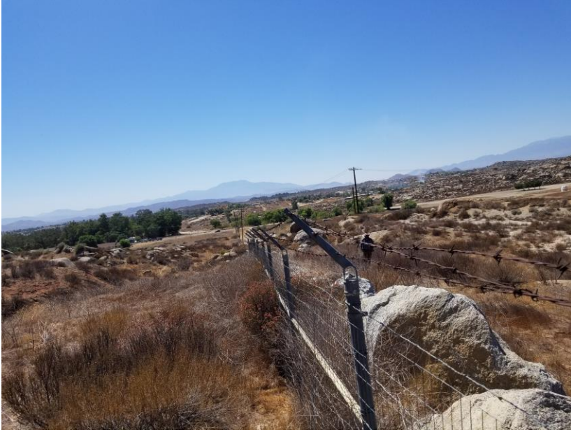
Photo 3: Existing Fence Overview (View NE)
