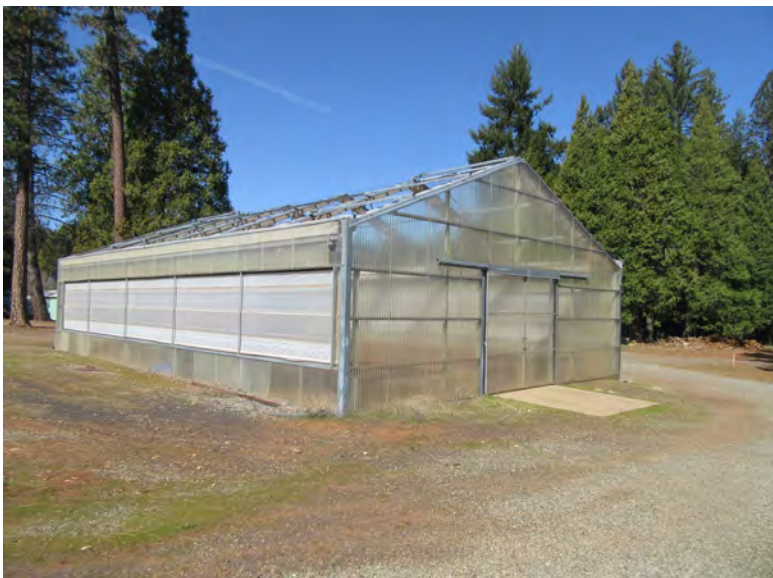
Existing greenhouse, to be demolished.
