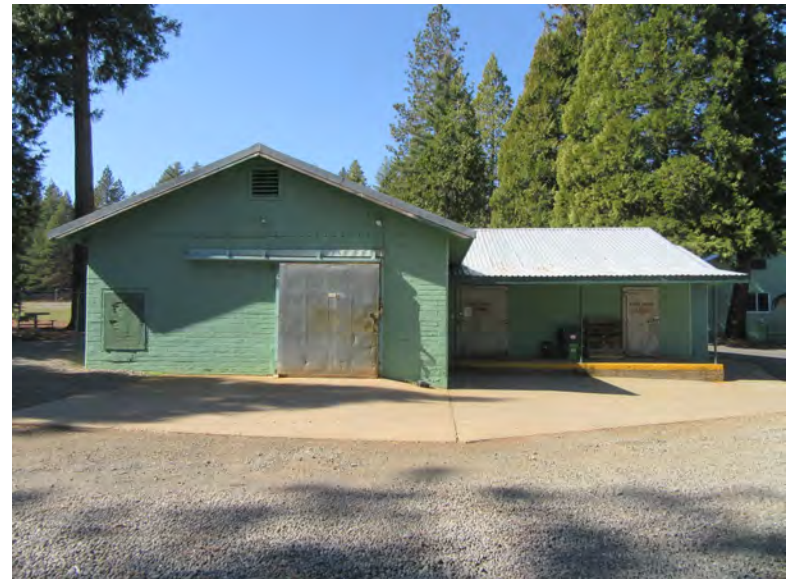
Existing refrigerated storage building, to be demolished.
