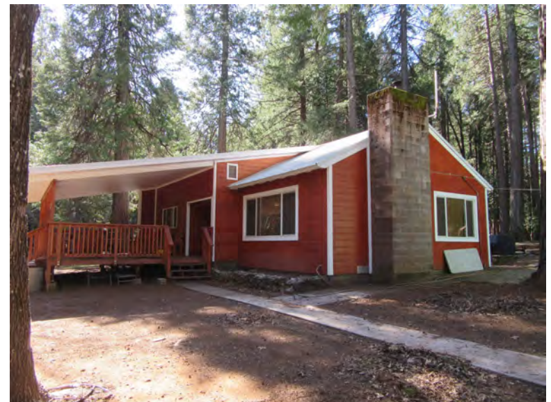
Existing captain's barracks, to be demolished.
