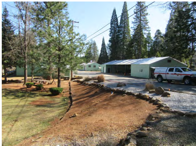
Looking east down Steiffer Road. Garages on south side of road would be demolished.
