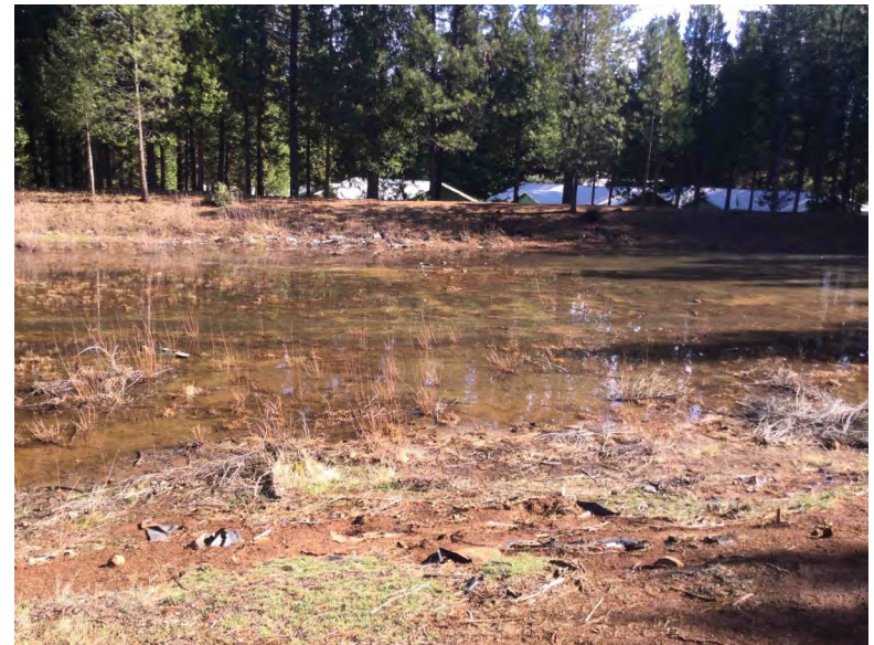
Looking east toward existing retention basin.
