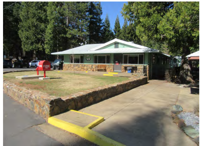
Existing CCC administration building, to be demolished.
